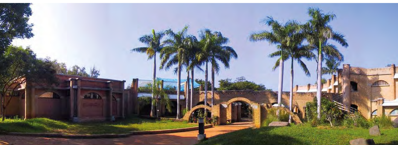
Figure 164—Visitor's Centre, Auroville, India (Photo credits: Satprem Maini)
