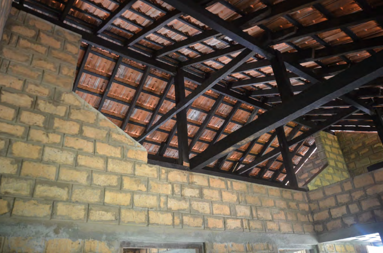
Figure 108—Roof truss and internal buttressing allowing for ventilation in Theravil Kulam, Mullaitivu district, built with the assistance of HfH and funded by the EU. (Source: Jaime Royo-Olid, EU 2018)
