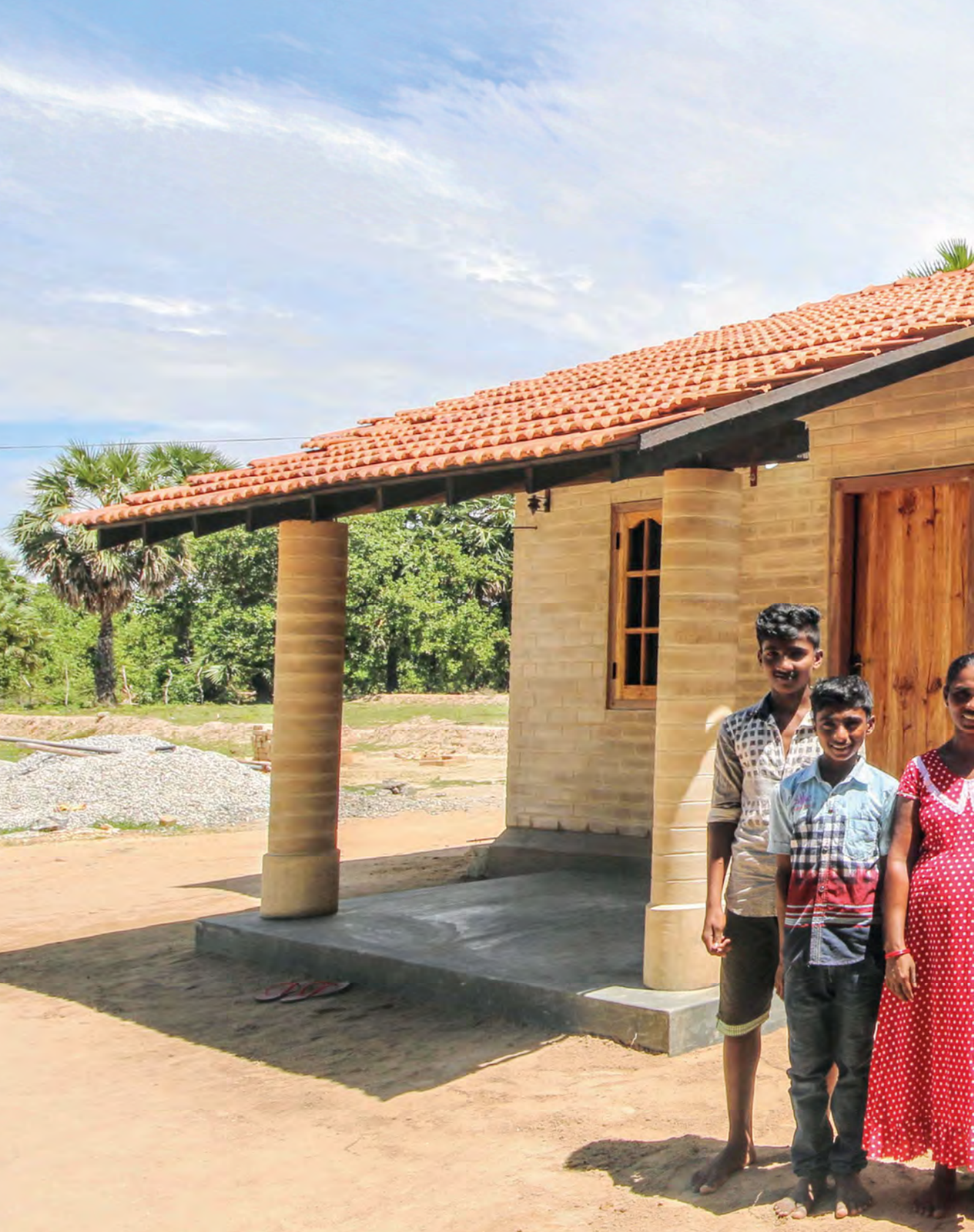
Figure 38—Family posing in front of their Compressed Stabilised Earth Block model house in Batticaloa built by Habitat for Humanity with the technical assistance and design of the directors of the Auroville Earth Institute for EUR 4 000. Funded by the EU. (Source: Satprem Maïni, 2017)
