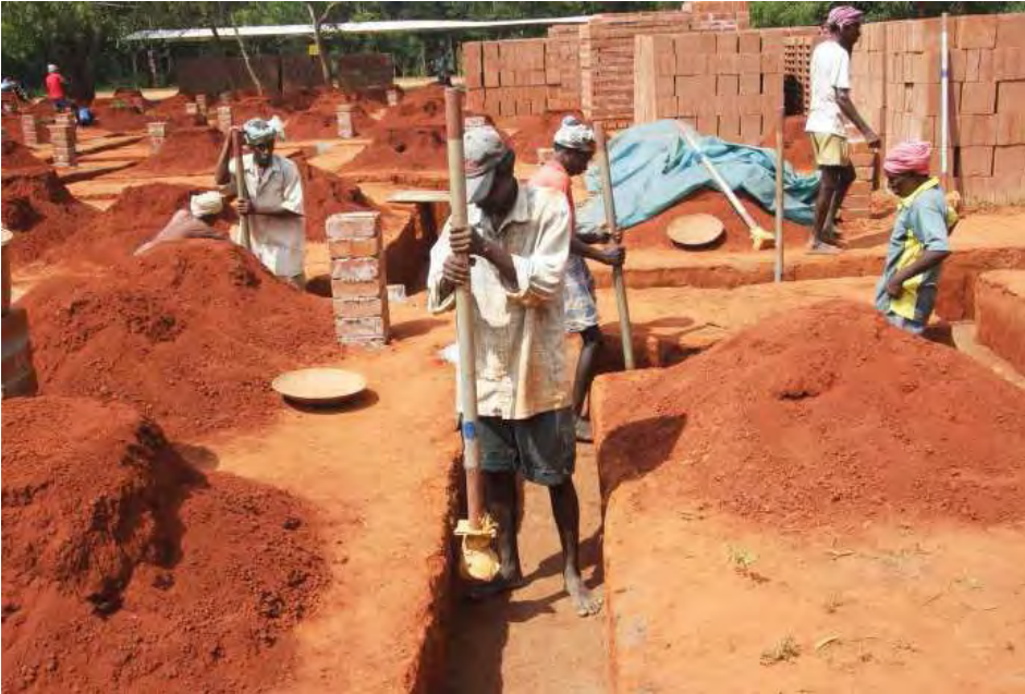
Figure 151—Ramming stabilised rammed earth foundations (Photo: Satprem Maïni)
