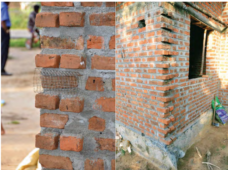
Figure 28—Protrusions to facilitate future extension of external walls made of conventional country-fired brick wall. Funded by the EU and implemented by Habitat for Humanity in Batticaloa (Source: Jaime Royo-Oluid, EU 2017)
