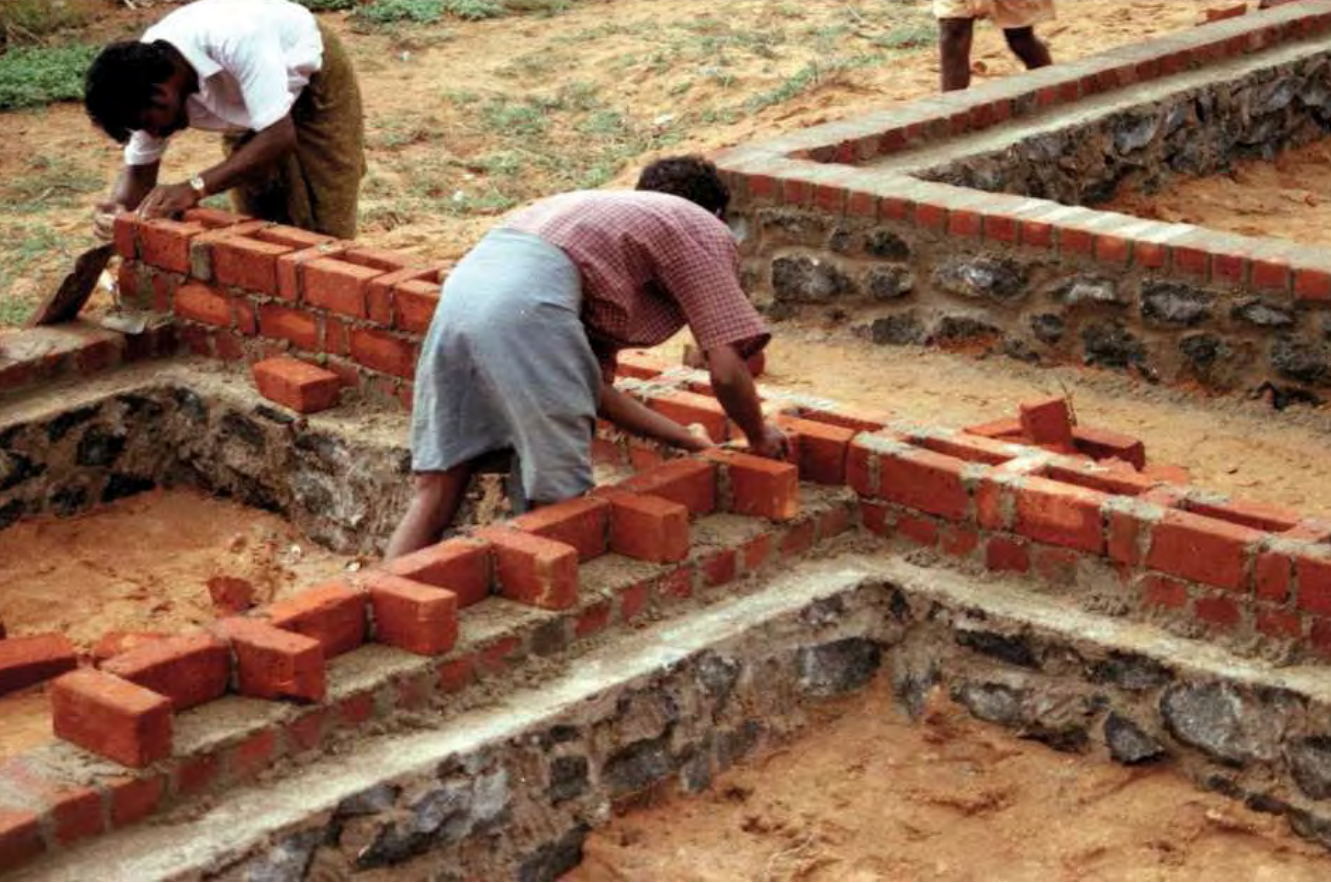
Figure 63—HTG head masons and local community trainee build post-tsunami house with rat-trap bond over local granite foundation. (Photo: Jaime Royo Olid, 2005)
