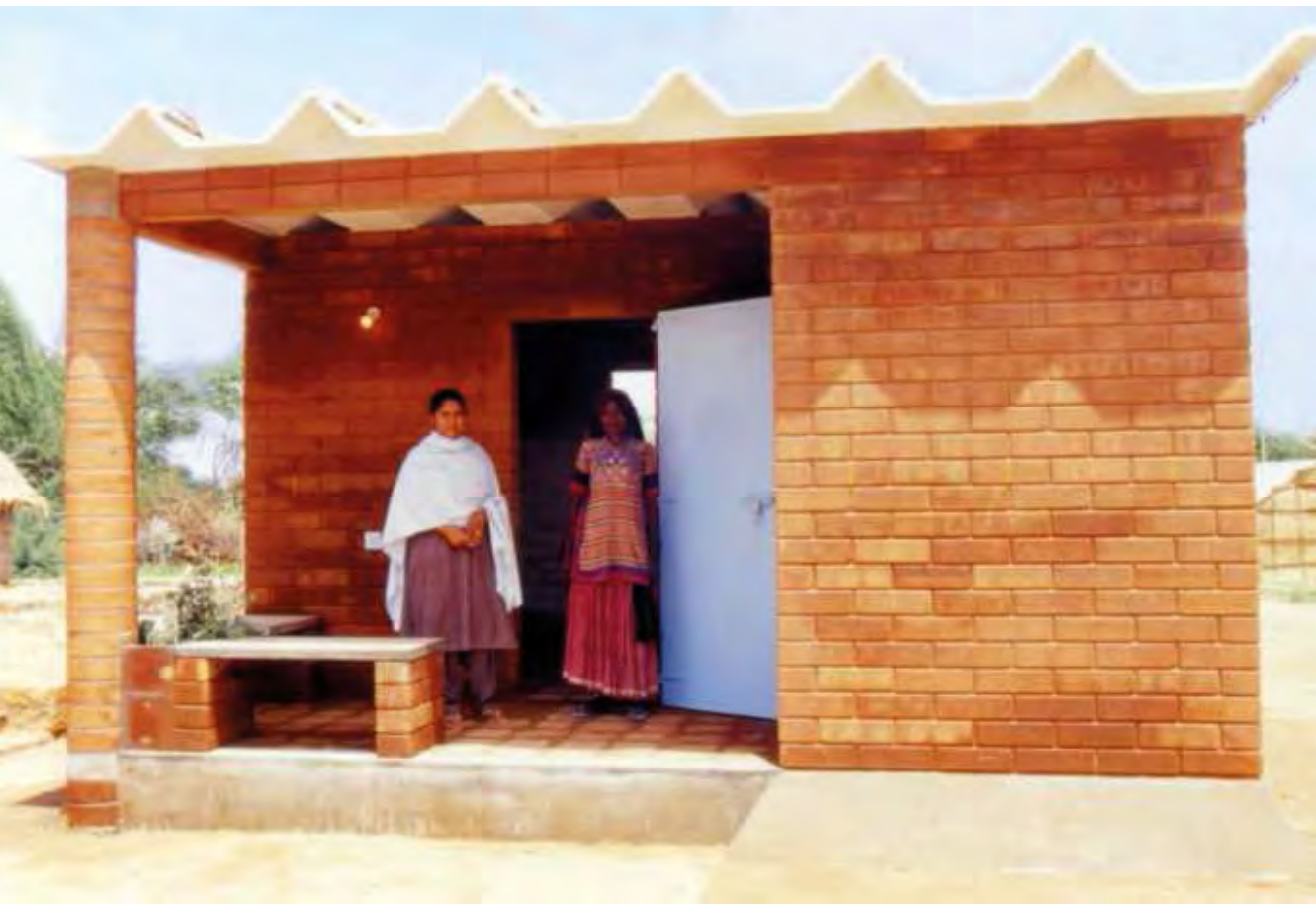
Figure 161—‘Aum House’ built in 62 hours, Gujarat, India (Photo: Satprem Maini)
