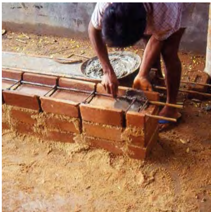
Figure 159—Composite lintel triple height, (Photo: Satprem Maini)
