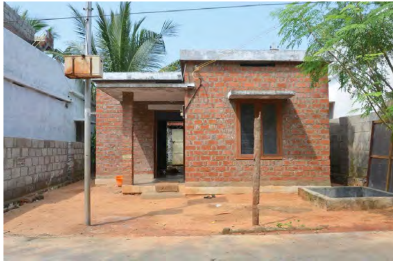
Figure 69—Above: Original house type unchanged in 2013. Exposed rat-trap bond and filler slab. Below: Same house-type after various vertical and horizontal expansions. (Photos: Jaime Royo-Olid, 2012)
