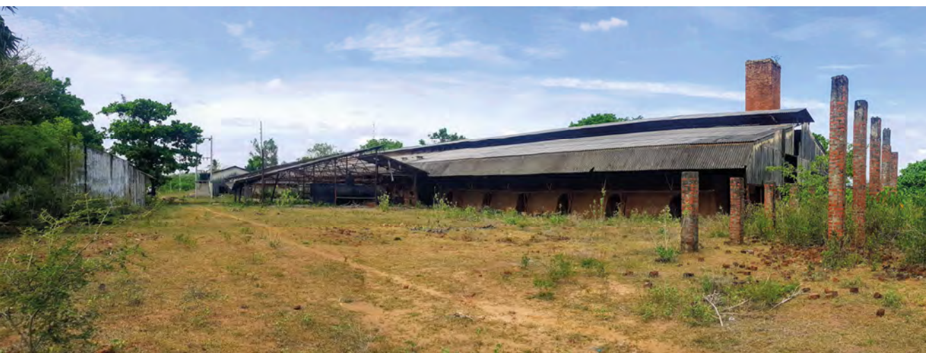
Figure 34—Abandoned tiles and brick factory in Uddusudan, Mullaitivu district, Sri Lanka (Source: Jaime Royo-Olid, EU 2018)
