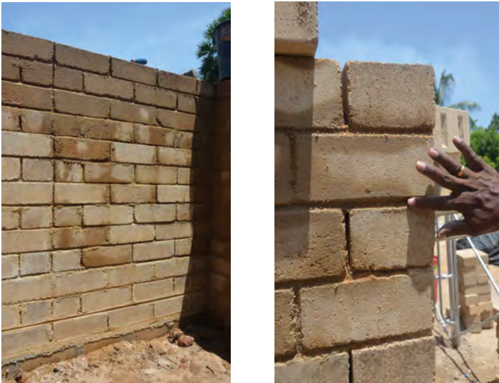
Figure 101—Joints of CSEBs prepared for future expansion. Left: for future doorway. Right: finger points sand (weak) mortar for easy extension of wall.
