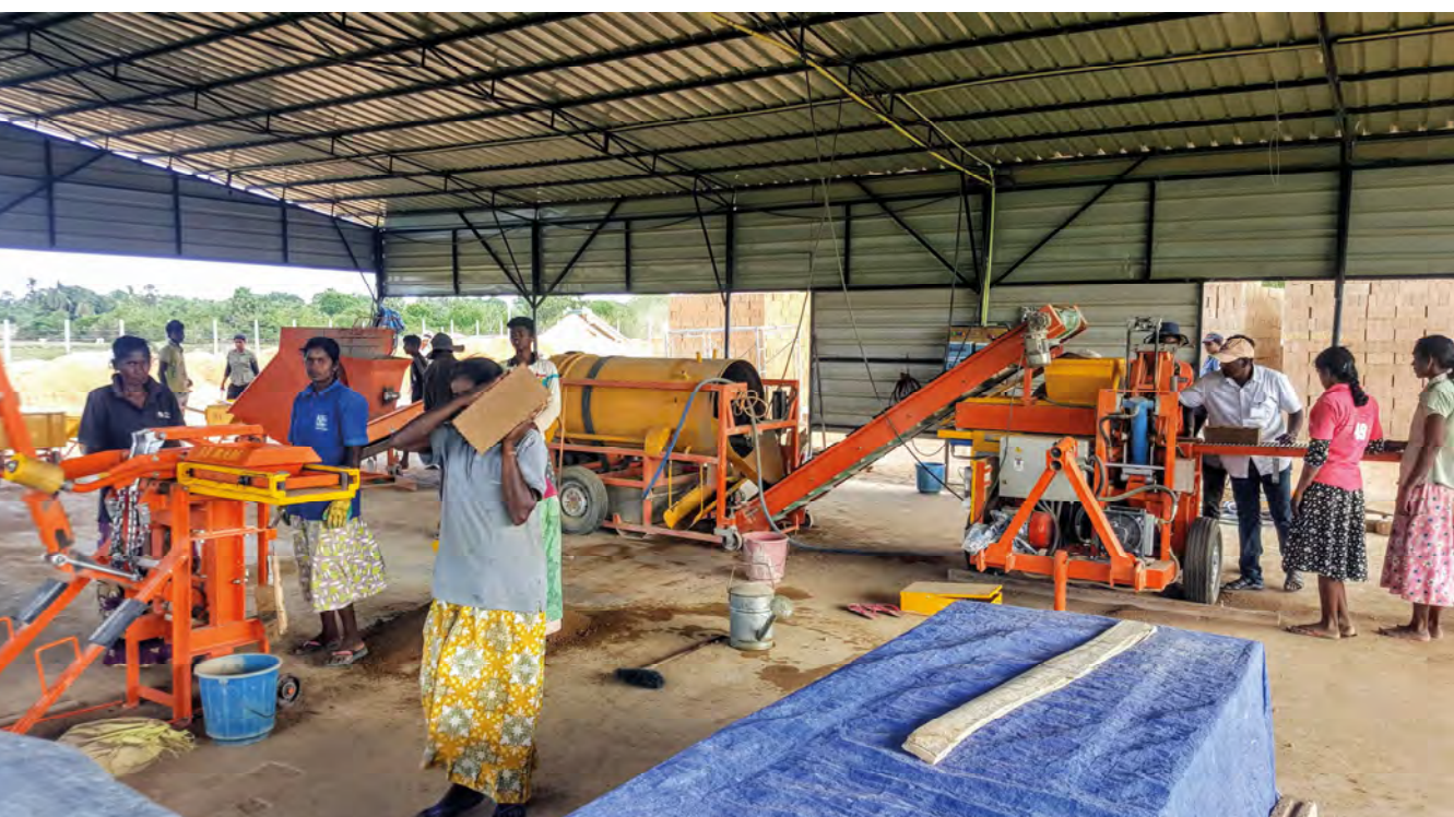
Figure 175—CSEB production yard in Batticaloa set up by HfHSL and WVJ with the technical assistance of the director of the Auroville Earth Institute. (Source: Jaime Royo-Olid, EU 2018)
