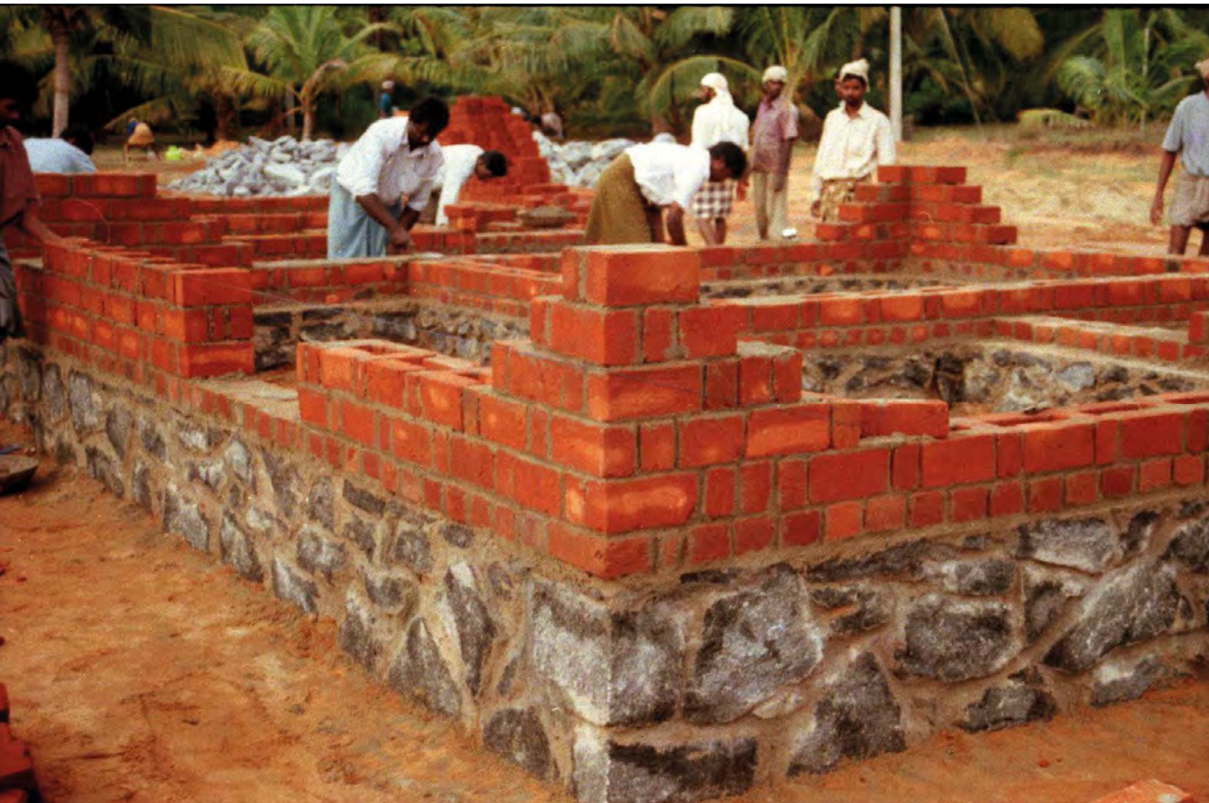
Figure 72—Veerapagupathi house construction in progress. Locally-sourced granite foundation and rat-trap bond brickwork being constructed by homeowners. (Source: Jaime Royo Olid, 2005)
