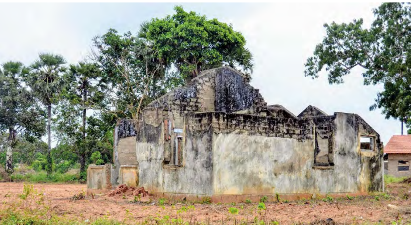
Figure 3—House destroyed during the conflict in Mannar District, Sri Lanka (Source: Jaime Royo-Oluid, EU 2013)
