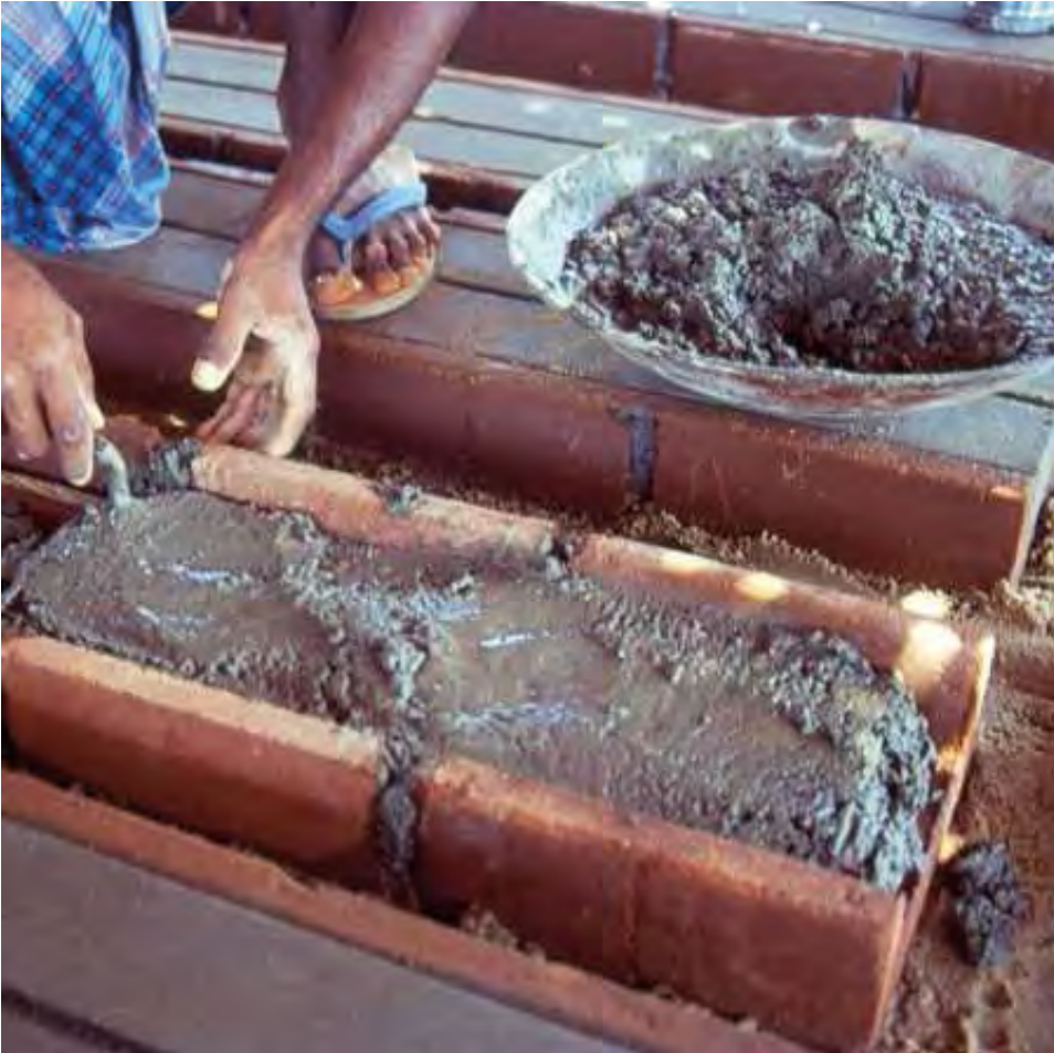
Figure 157—Composite lintel-single height, (Photo: Satprem Mañi)
