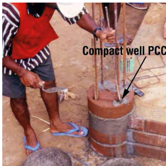
Figure 155—Composite column 290, (Photo: Satprem Maïni)
