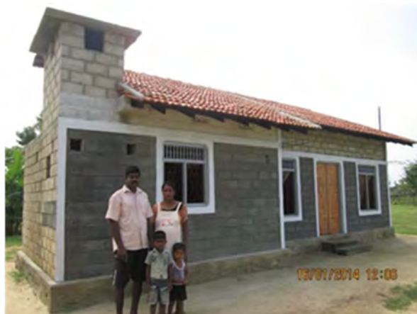
Figure 122—House built with fair-face technology which saves plaster, sand, cement, lime and labour (Source: UN-Habitat 2014)
