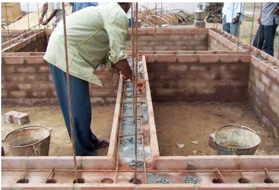
Figure 160—Reinforced masonry with hollow interlocking CSEB (Photo: Satprem Maïni)
