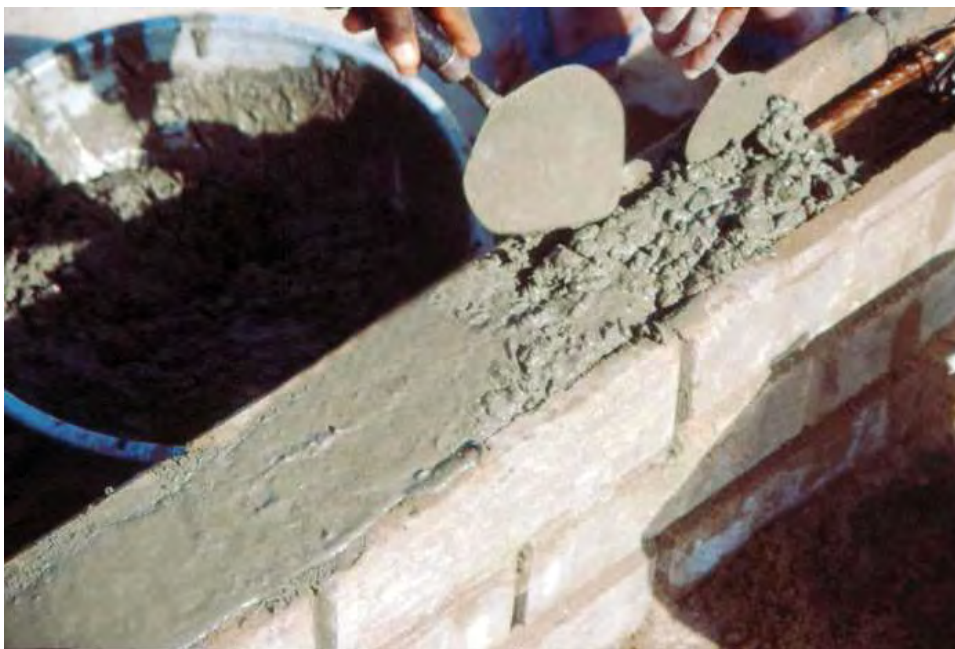
Figure 153—Casting a composite plinth beam (Photo: Satprem Mañni)
