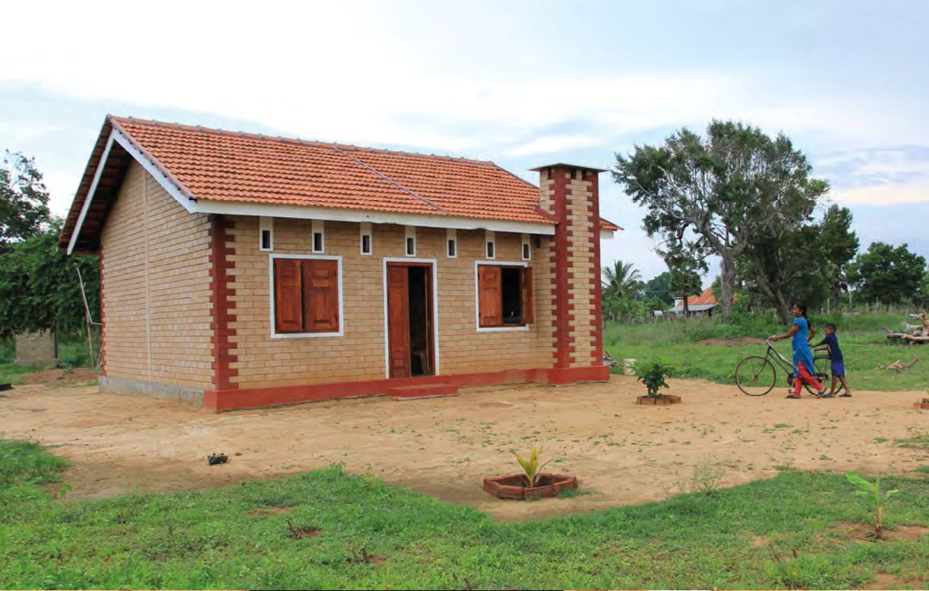
Figure 120—Model house owned by Ms Vasuki built with interlocking CSEB under the IHP (Source: UN-Habitat, 2014)
