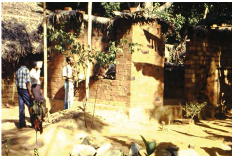
Figure 21—Example of incremental house built under the MHP in 1986 where the owner run out of financial and material resources to complete overambitious house.
