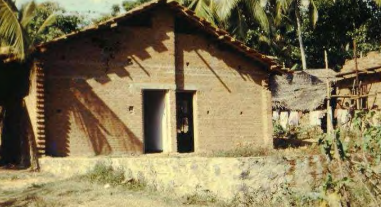
Figure 11—Incremental House built under the Million Houses Programme (MHP) with foundation ready for future expansion. (Source: Dr Mano Kumarasuriyar, Mid-term Evaluation 1986-87)
