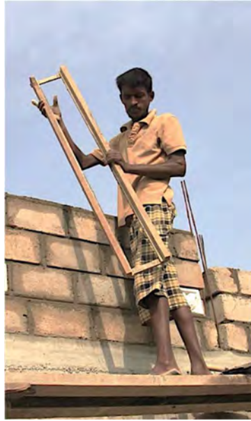
Figure 123—New tools in fair-face block work. Traditional mason first feels insecure until they witness the outcome. (Source: UN-Habitat 2014)
