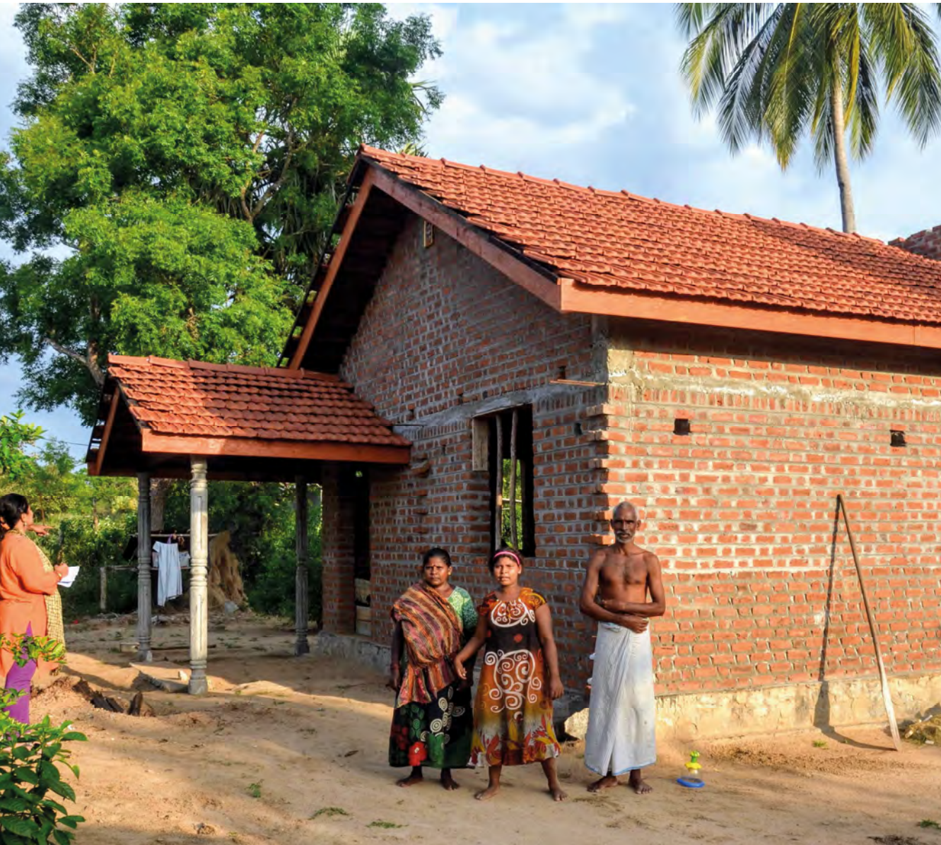
Figure 29—EU-funded owner-driven house built with the assistance of Habitat for Humanity, Batticaloa. (Photo: Jaime Royo-Olid, EU 2017)
