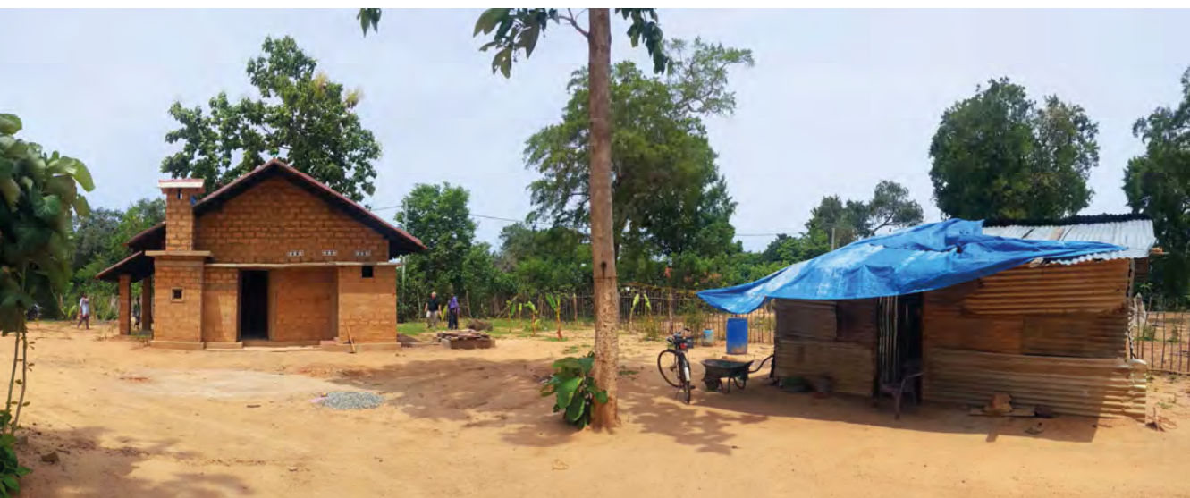
Figure 1—Left, EU-funded model house built by the owners with locally-sourced Earth Concrete Blocks with the assistance of Habitat for Humanity Sri Lanka in Batticaloa, Sri Lanka. Right, shelter where family has been living for almost a decade. (Source: Jaime Royo-Olid, EU 2018)
