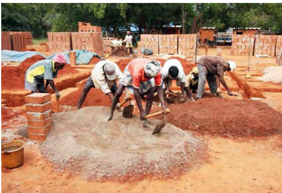
Figure 150—Mixing for a stabilised rammed earth foundation
