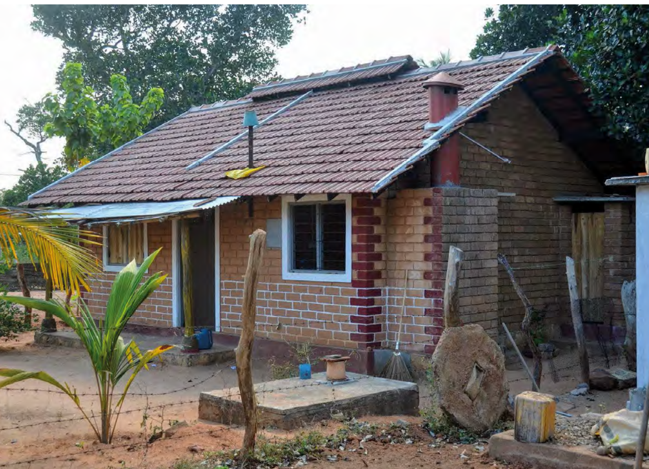
Figure 127—EU-funded model house built with the assistance of UN-Habitat using interlocking CSEB in Mullaitivu District (Photo: Jaime Royo-Oluid, EU 2016).
