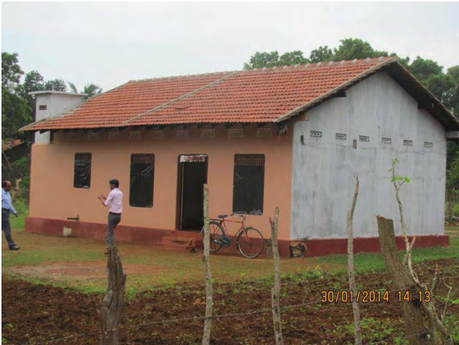
Figure 94—Even a 550 sq. ft. house is not big enough; most families contributed own savings for a bigger space and higher specifications (Photo: Kirtee Shah)
