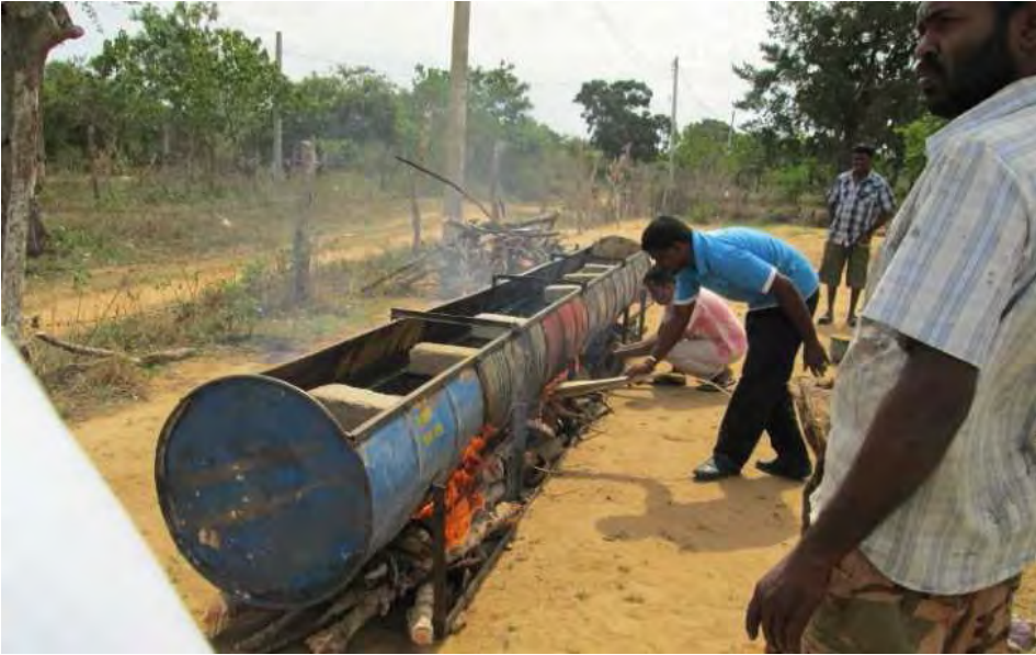
Figure 125—On-site treating of plantation timber using engine oil. (Source: UN-Habitat 2014)
