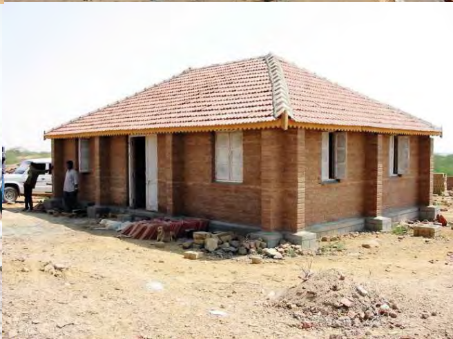
Figure 172—Two million CSEB produced for the construction of 2 698 Houses in 1 year, Gujarat, India (Photo: CRS)
