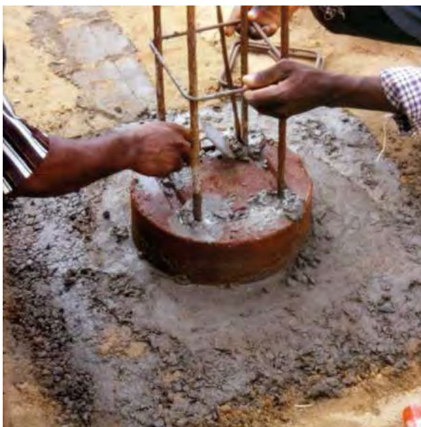
Figure 154—Composite column 240, (Photo: Satprem Maïni)
