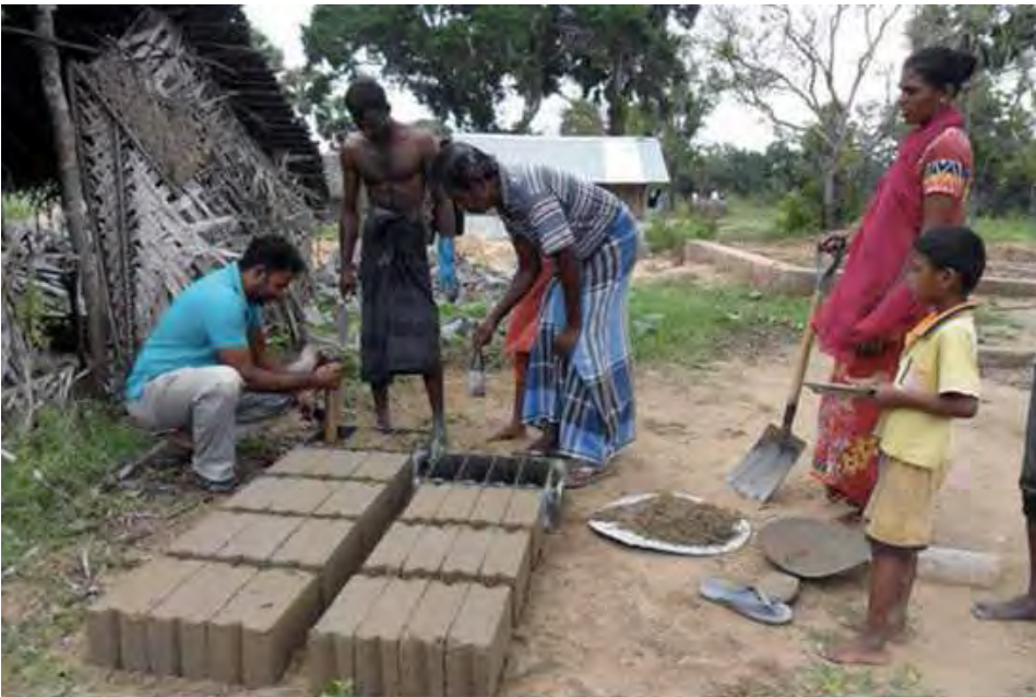
Figure 119—Cement-block making advice and training being provided by UN-Habitat to homeowner, S. A. Kafoor in Karadikkuli, Musali DS division Mannar. (Copyright: Ms Ubaitullah, UN-Habitat, 2013)
