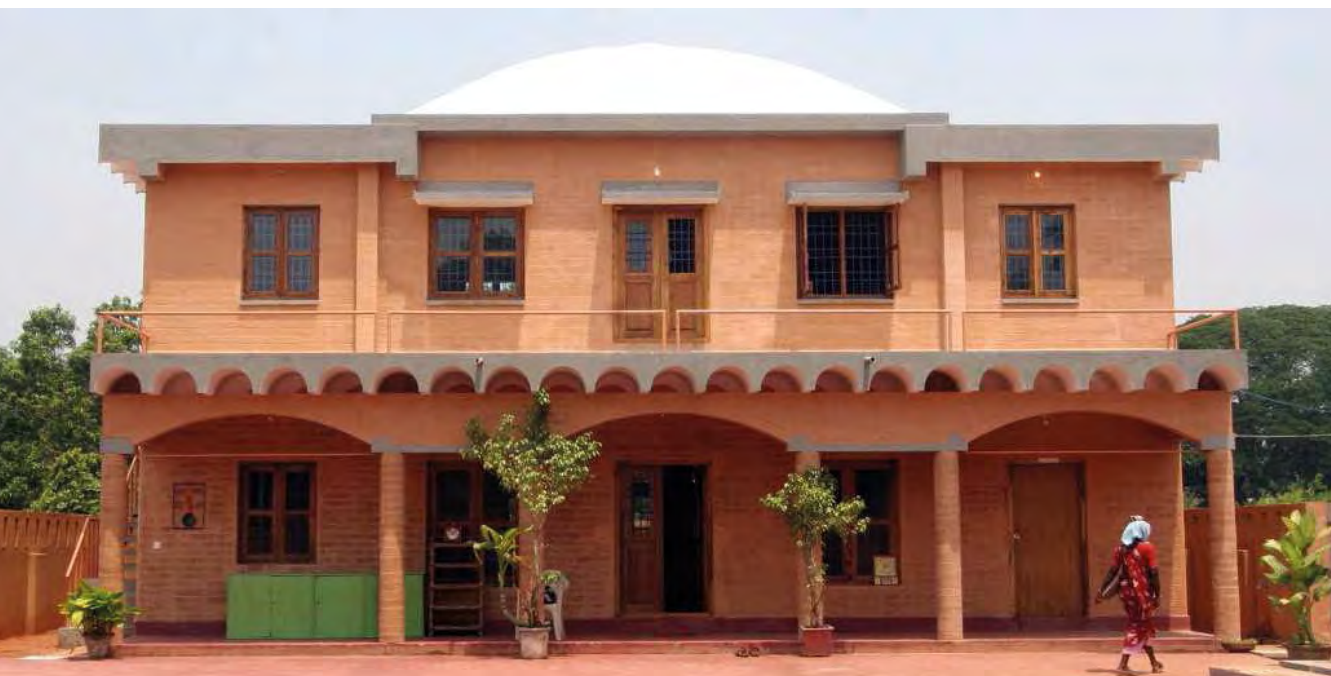
Figure 167—Marakkanam School & Community centre, Marakkanam, India (Photo: Satprem Māini)
