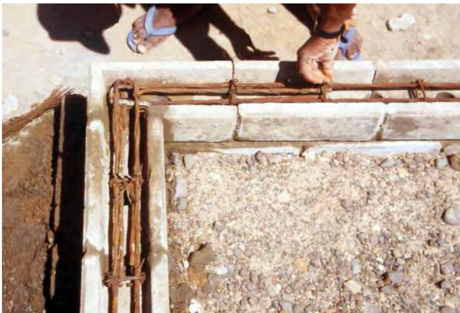
Figure 152—Composite plinth beam (Photo: Satprem Mañni)
