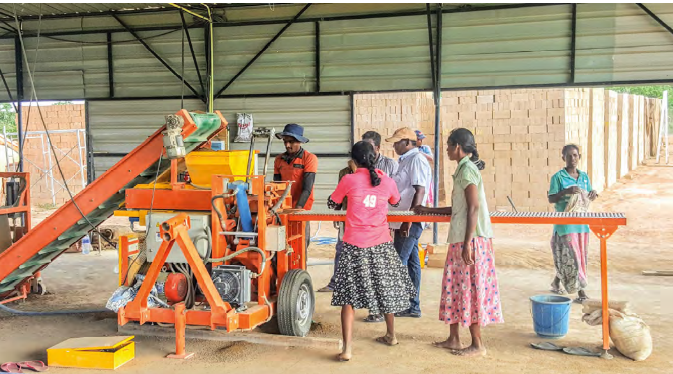
Figure 35—CSEB production yard established by HfHSL and WV in Baticaloa funded by the EU (Source: Jaime Royo-Olid, EU 2017)
