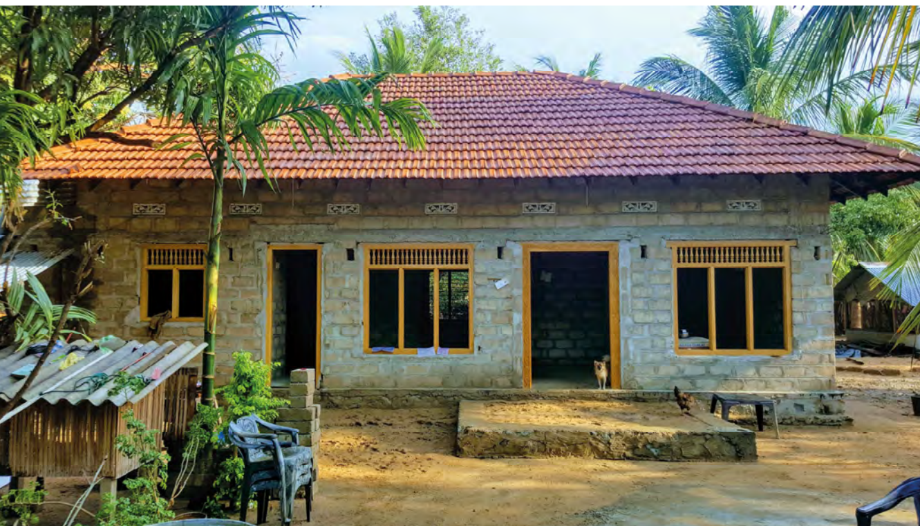
Figure 98—Self-built 900 sq. ft house in Kilinochchi by HfH beneficiary homeowner beyond NERHP standards using cement sand blocks. This house symbolises the post-reconstruction aspirations of resettled communities. (Source: Jaime Royo-Olid, EU 2017)
