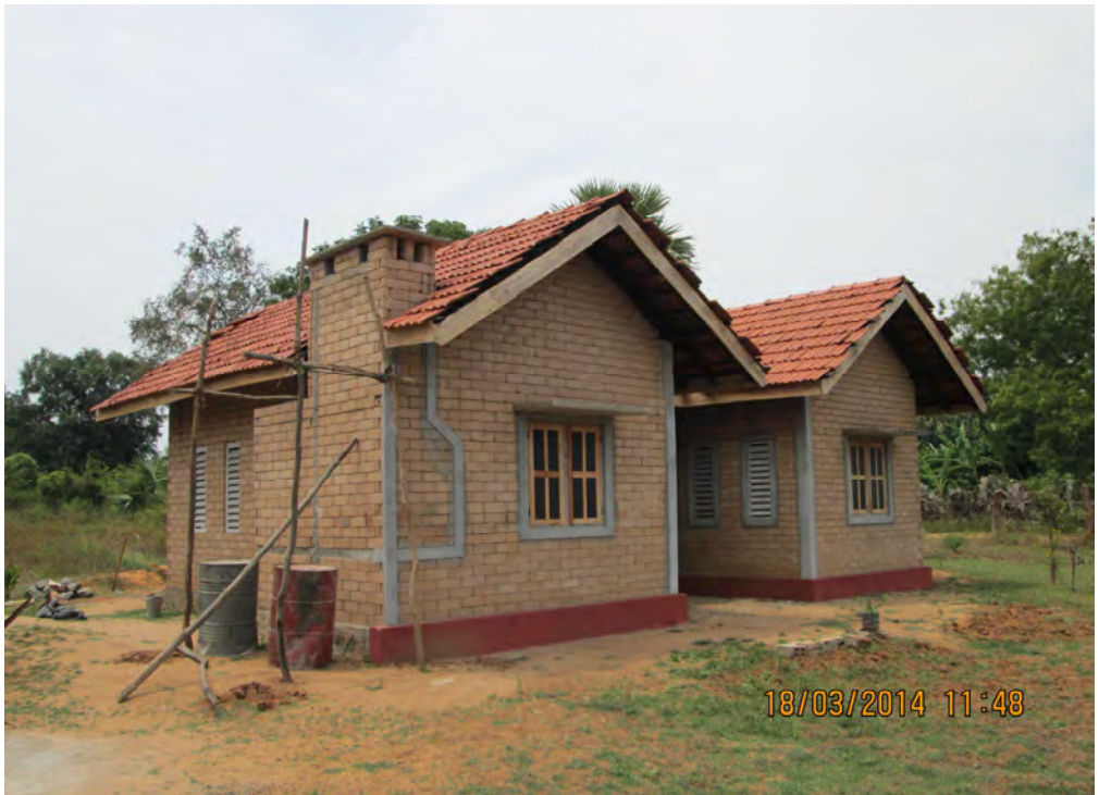
Figure 124—Experimental model U-shaped house (not replicated) built with interlocking CSEB under the IHP (Source: UN-Habitat, 2014)
