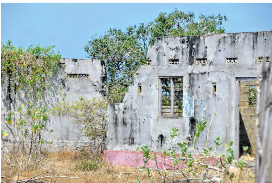
Figure 214—House ruined by conflict in Millivaikal, Mullaitivu district, Sri Lanka (Photo: Jaime Royo-Olid, EU 2016)
