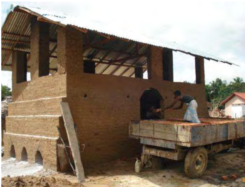
Figure 186—Improved brick kiln in eastern province (Source: Practical Action)
