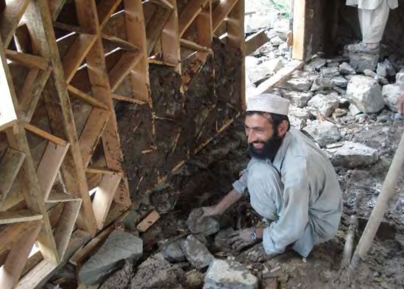
Figure 14 Rebuilding with earthquake-resistant traditional technology (Dhaji) in Pakistan, 2007 (Source: UN-Habitat)
