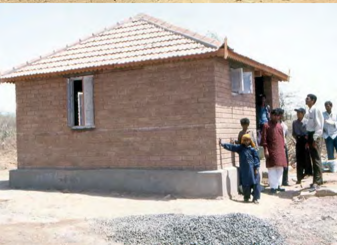
Figure 172—Two million CSEB produced for the construction of 2 698 Houses in 1 year, Gujarat, India (Photo: CRS)
