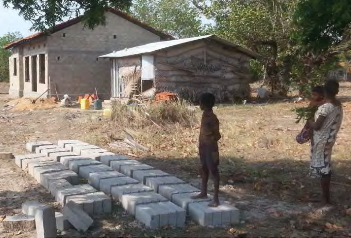
Figure 196—From temporary shelter to permanent housing: child from resettled family observes progress on the house being built through owner-driven-assistance by his family next to the temporary shack they currently live in (Photo: SDC)
