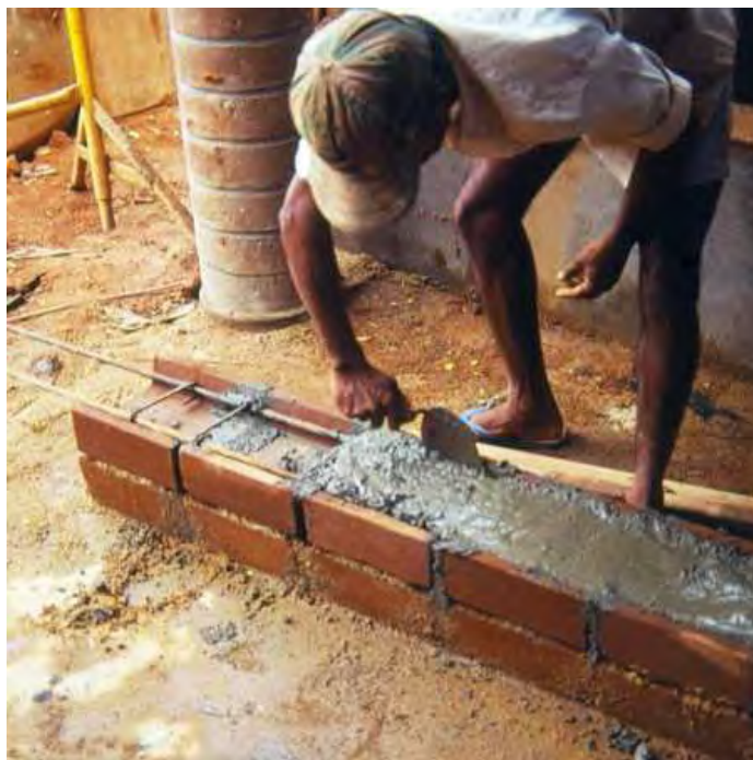
Figure 158—Composite lintel-double height, (Photo: Satprem Maini)
