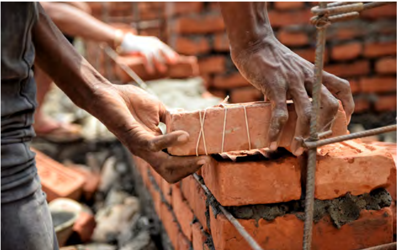
Fig. 3: © Bria Fast, Nepal, 2016. A mason lays bricks during reconstruction of a home after the Nepal earthquake.
