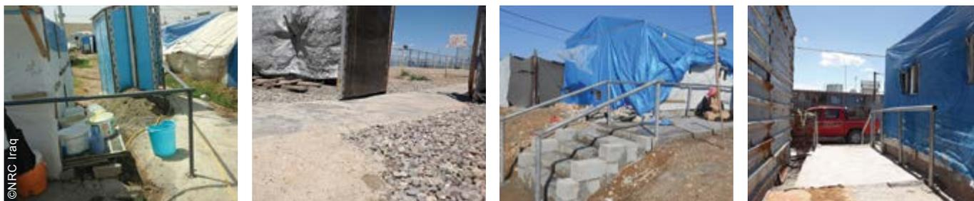
Works also included mobility upgrades within plots or across the camps. From left to right: Concrete pathway and railing leading from shelter to shared/communal latrine. Concrete slab improving wheelchair access. Handrails, concrete stairway and pathway around or between shelter plots.
