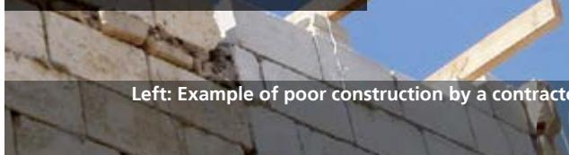
Left: Example of poor construction by a contractor in 2007, Wooden girders insufficient to support the new roof.
