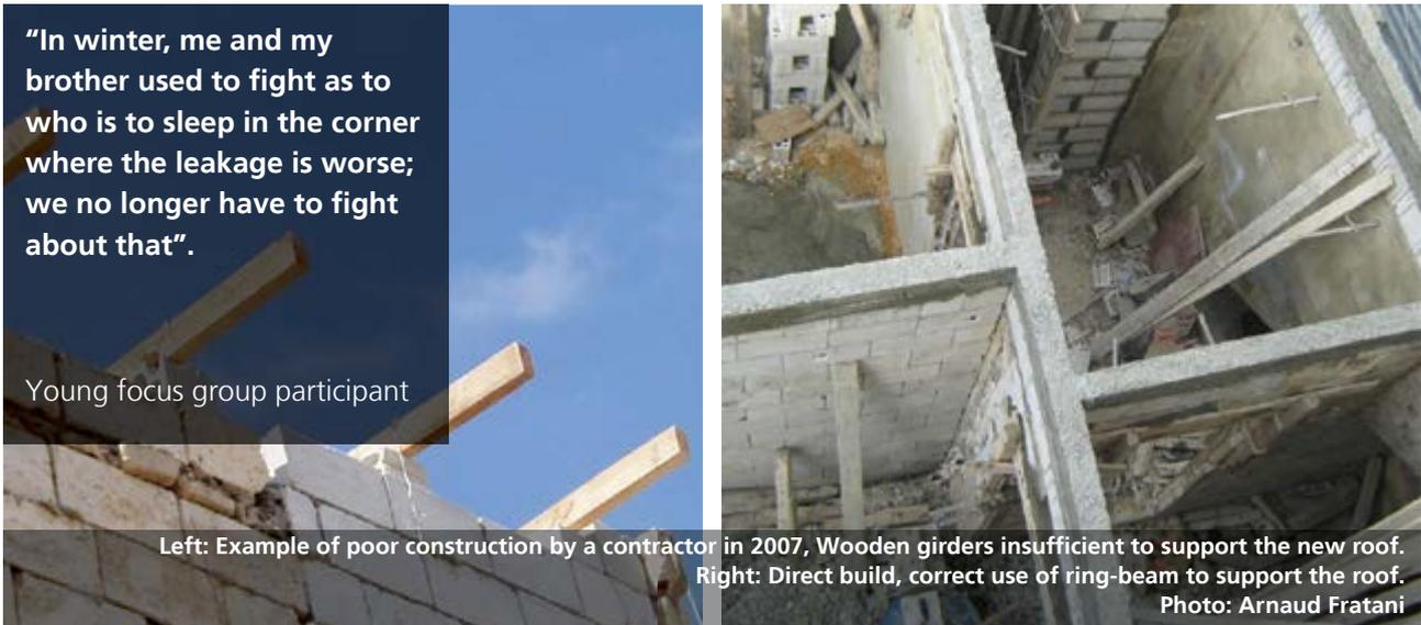
Left: Example of poor construction by a contractor in 2007, Wooden girders insufficient to support the new roof. Right: Direct build, correct use of ring-beam to support the roof. Photo: Arnaud Fratani
