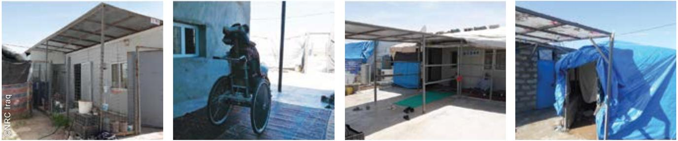
The project worked on a variety of upgrades focused on improving the accessibility and Quality of Life of individuals with disabilities. From left to right: Shaded area and fencing around prefab shelter. Concrete slab improving wheelchair access. Fold out support railing. Shaded entrance and support posts for better access.
