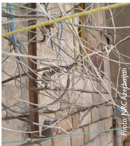
Wiring before upgrade
