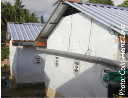
Shelters built with tanks for rainwater harvesting
