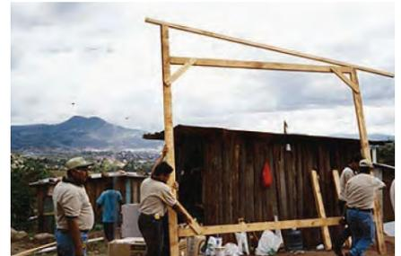
Shelter assembly using prefabricated walls
