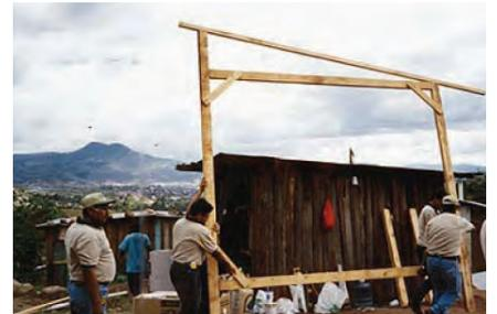
Shelter assembly using prefabricated walls
