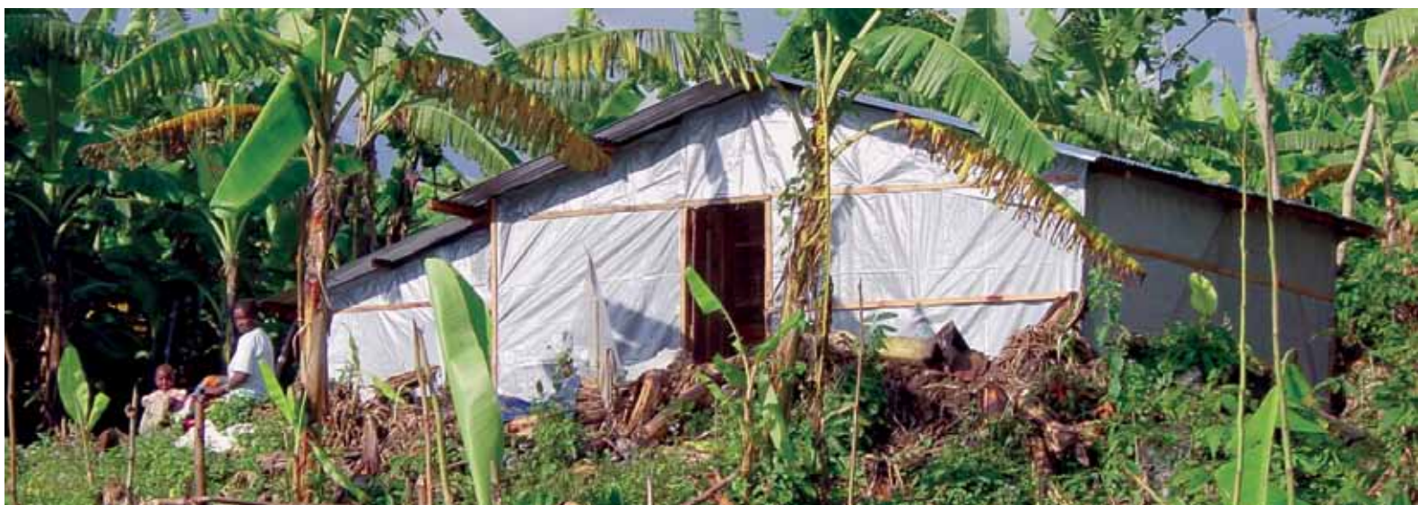
A temporary house built during this project Photo: Graham Saunders
