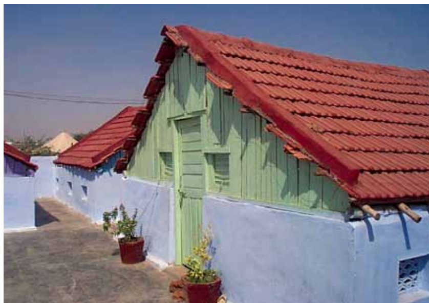
These school buildings were adapted from the transitional shelters. The low walls reduced the risk of masonry falling on occupants during future earthquakes. Photo: Chris Cattaway
