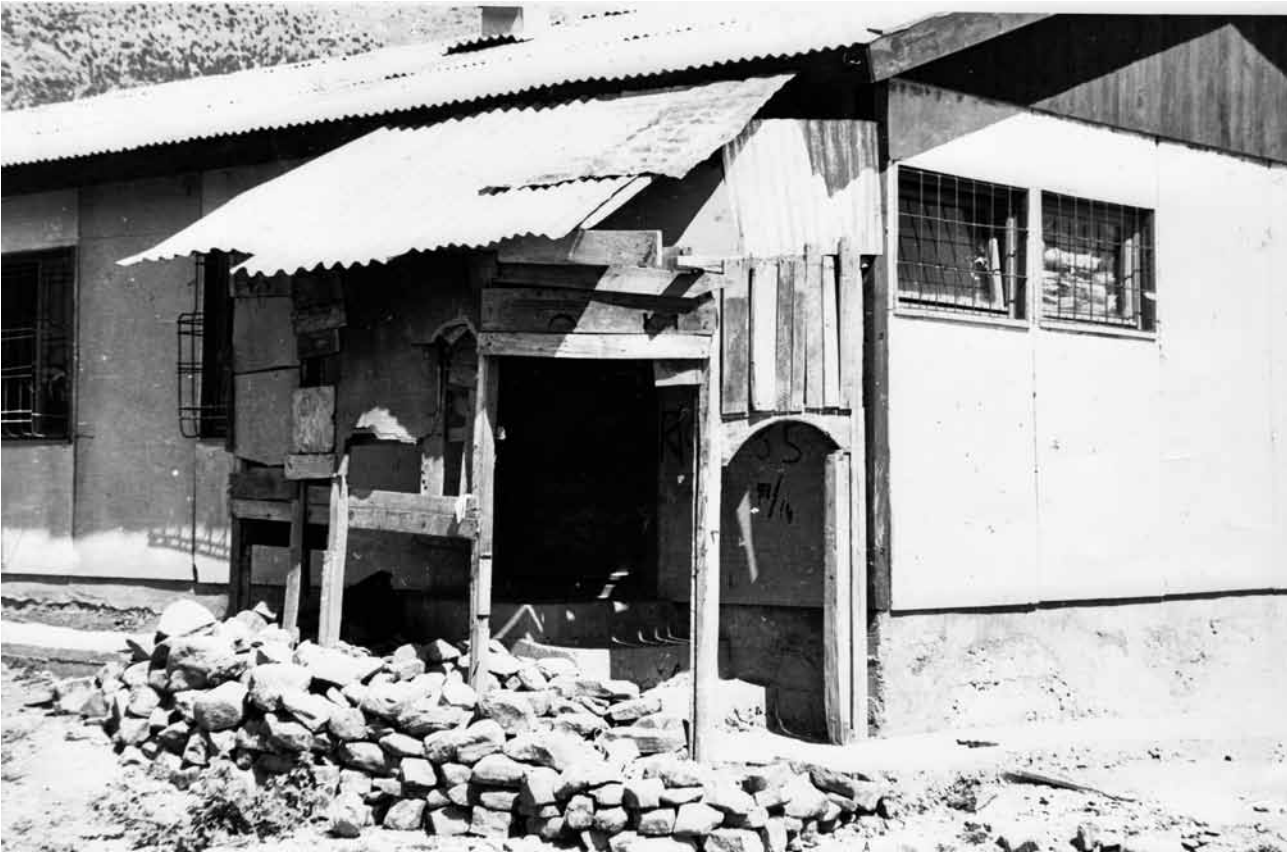
A family added this porch to their new prefabricated home. It is an example of the need for protection for an animal, and also some protection for the door. Photo: Ian Davis
