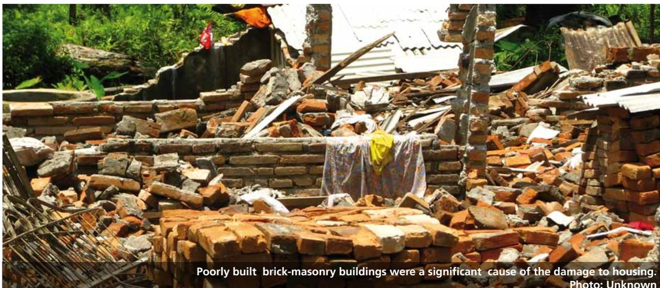
Poorly built brick-masonry buildings were a significant cause of the damage to housing. Photo: Unknown
