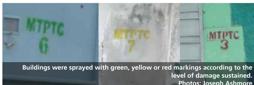
Buildings were sprayed with green, yellow or red markings according to the level of damage sustained.
