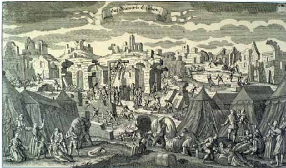
1755 German copperplate image, The Ruins of Lisbon: In the left of illustration is a tented camp in the suburbs of Lisbon following the fire of 1755. On the right damage that is probably related to the 1531 earthquake.
