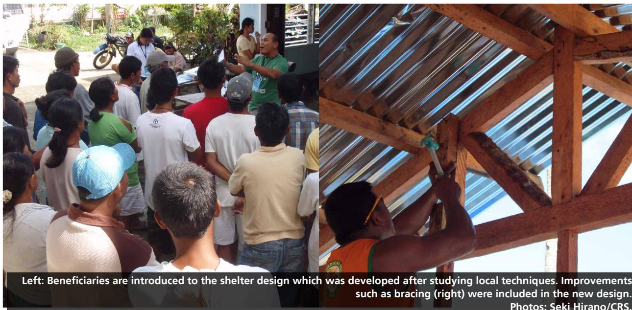
Left: Beneficiaries are introduced to the shelter design which was developed after studying local techniques. Improvements such as bracing (right) were included in the new design. Photos: Seki Hirano/CRS.
