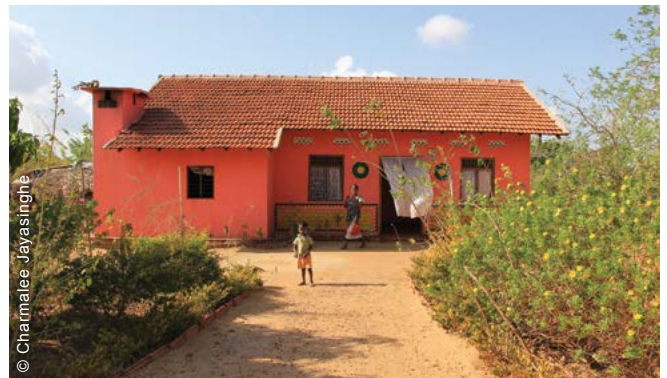
Completed house in Mullaitivu district. The use of reconstruction committees and community action planning methodologies helped restore social cohesion.
