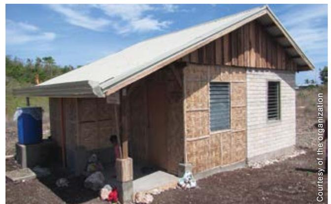
The project provided core houses with light-weight extensions, based on a common rural design. The houses included a gutter and a water tank for rainwater collection.
