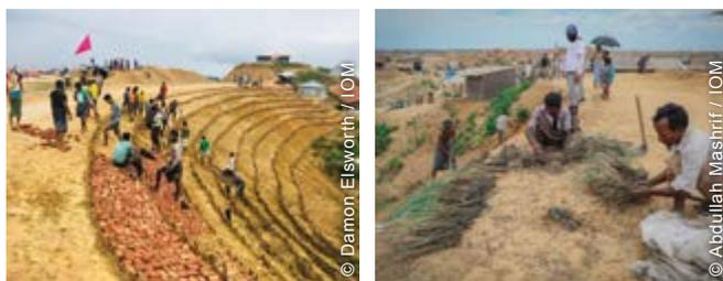
Site improvements were mainly conducted through cash for work and included slope protection by terracing (above-left) and vetiver plantation (above-right).
