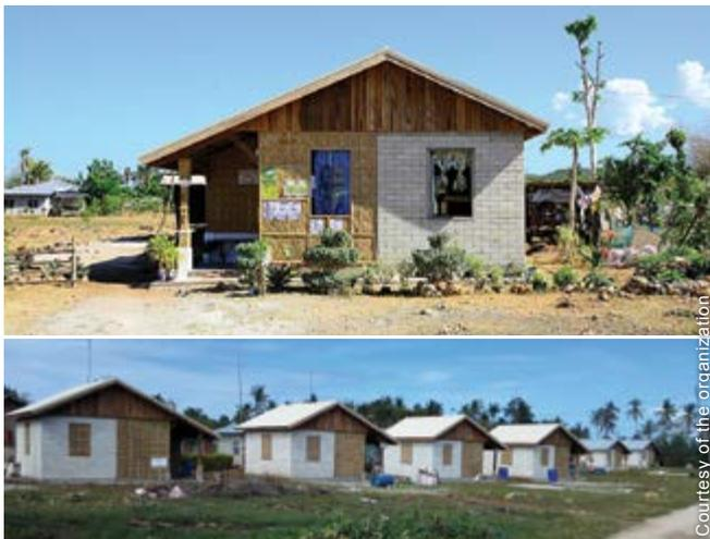
Core houses were built to resist typhoons and earthquakes and have an expected lifespan of 20 years for the core and 10 for the extension.
