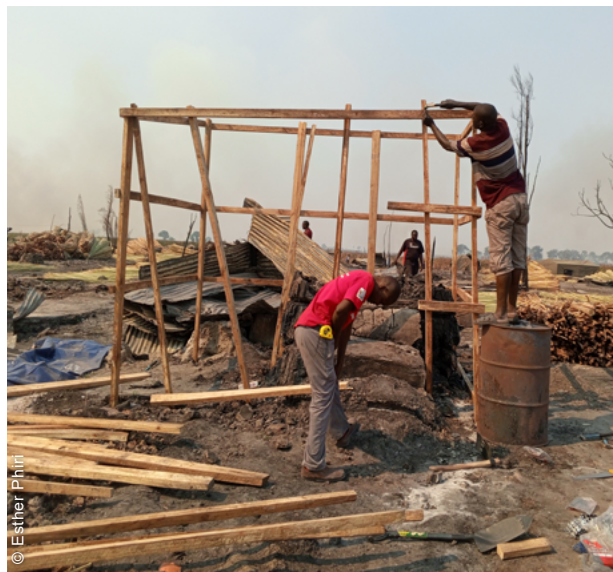
Building elevated toilets and bathing shelters in a burned down fishing village on the Kafue River, Zambia.
