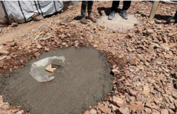
B - Concrete foundation pockets/slabs
