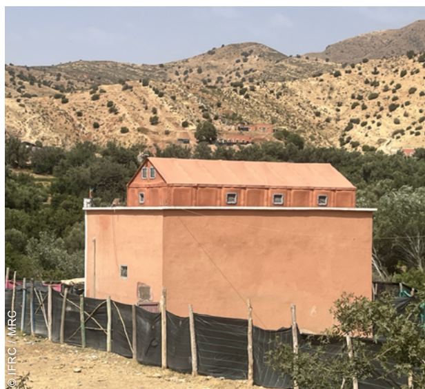
After repairing their houses, many people repurposed the TSUs, including as house extensions, or for storage.
