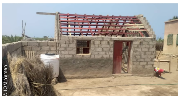
Some families used the cash to rebuild their roofs and complete their shelters.
