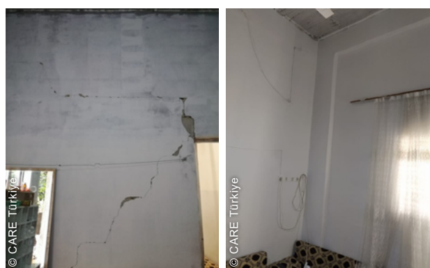
The project rehabilitated homes with light interventions such as covering cracks and repainting, particularly targeting vulnerable households.
