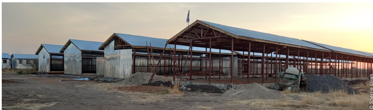
Semi-permanent communal shelters were constructed alongside basic facilities and clearly organized areas in the site.
