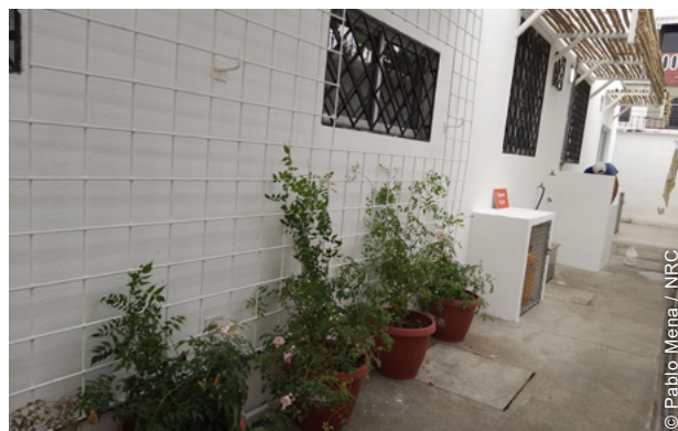
Interventions such as shading devices and green walls were implemented across six communal shelters, improving thermal comfort and reducing sun exposure.
