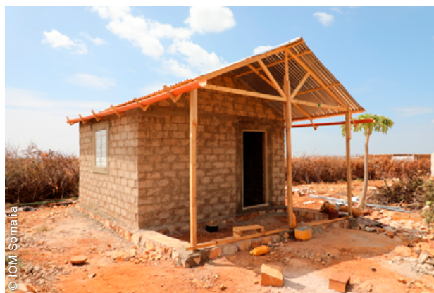
The most vulnerable households in the site received cement blocks shelters.
