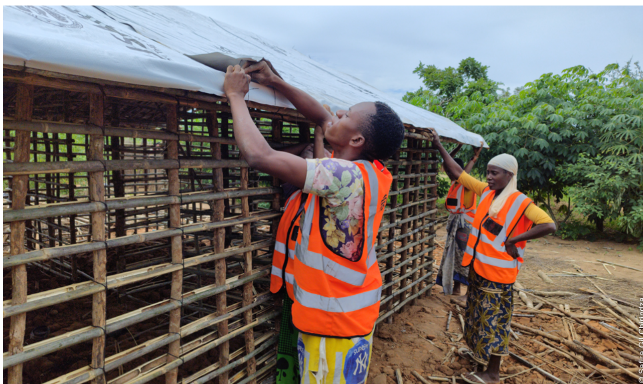
Build Back Better trainings strengthened household skills and introduced improved, resilient construction techniques aligned with local customs and traditional shelter models.
