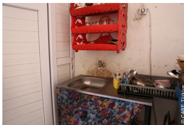
Sources of leaks and humidity, as well as external insulation, were addressed by the renovation interventions, to improve living conditions.
