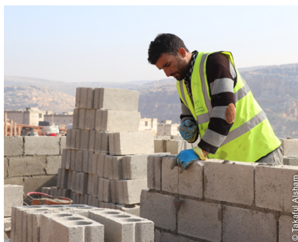
Shelter units and sanitation blocks were installed following site preparations.
