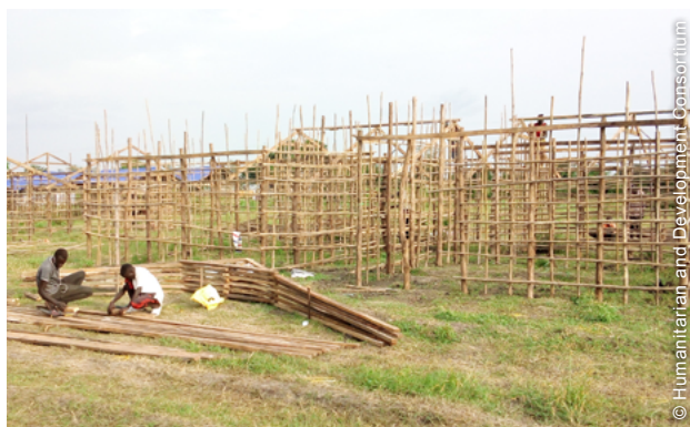
Materials for the shelter frames were procured from the Common Pipeline, while roofing sheets and hardware items came from local contractors.
