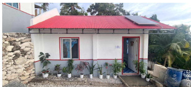
Solar panels were also installed to ensure energy supply in areas with limited electricity infrastructure.
