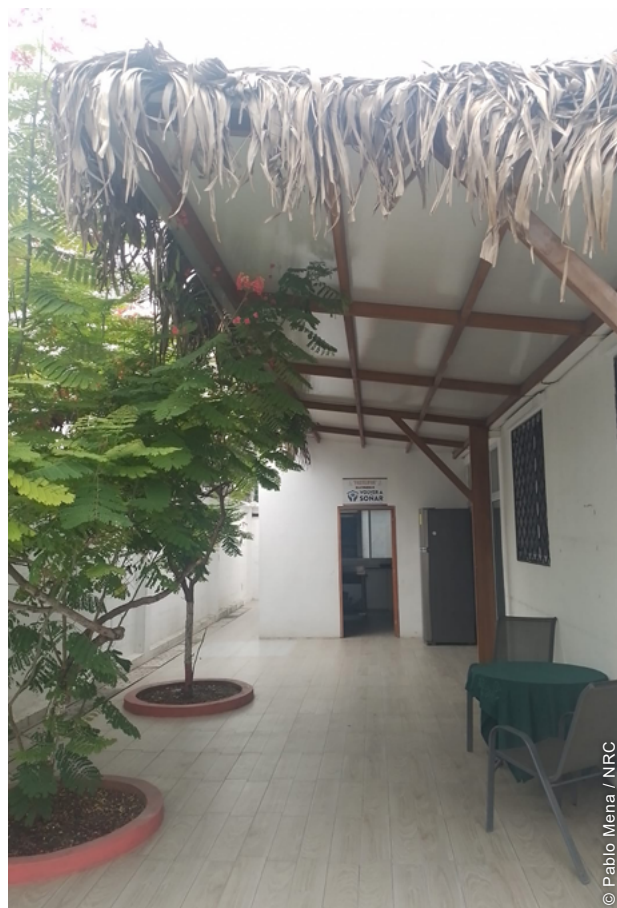
Using a direct implementation approach, shading devices and green elements were included to mitigate climate effects and increase comfort for the users.
