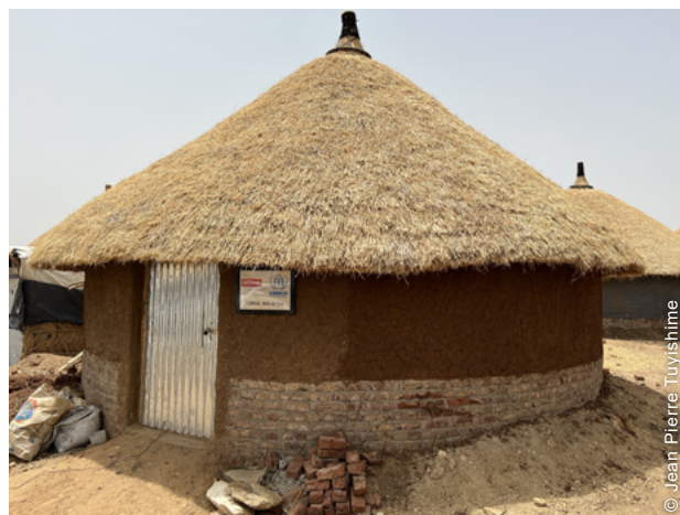
The project adopted locally accepted construction typologies, the tukuls, built with local materials and adapted to the climate.
