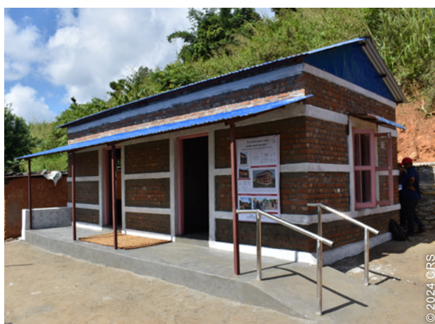
Ramps, handrails and accessible sanitation facilities were provided when needed by participants with disabilities.
