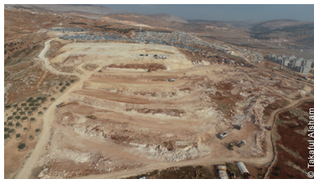
The project commenced with large grading and levelling works.
