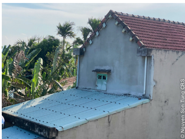
Roof escapes were created to allow quick exit during heavy floods.
