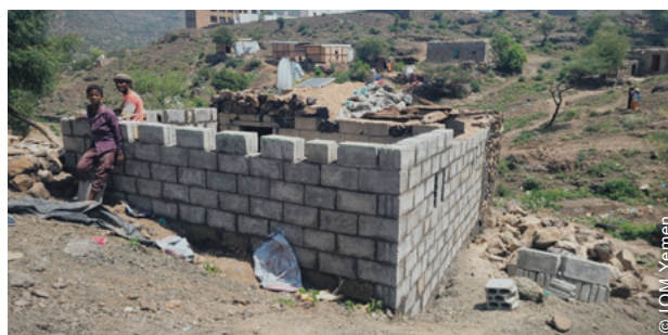
In other locations, households opted to rebuild or complete their unfinished structures using concrete blocks available in the local market.
