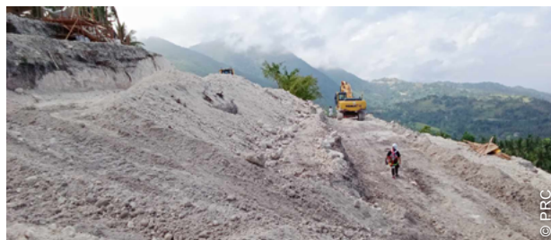
Site preparations were underestimated and required several adjustments.
