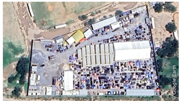
The photos show the site in the early stages of the centre (above, July 2022) and after the construction of the timber shelters (below, April 2023).
