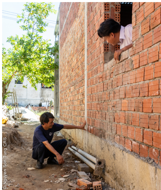
Raised foundations were built to reduce future flooding risks.
