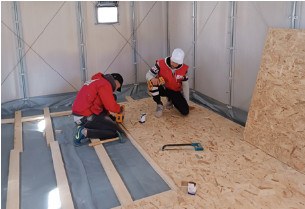
D - Installation of OSB wooden flooring platforms
