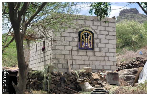
Windows and doors were installed thanks to the assistance received.
