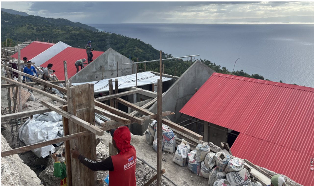
Permanent houses and site infrastructure were built on a slopy site using locally procured resources and labour.
