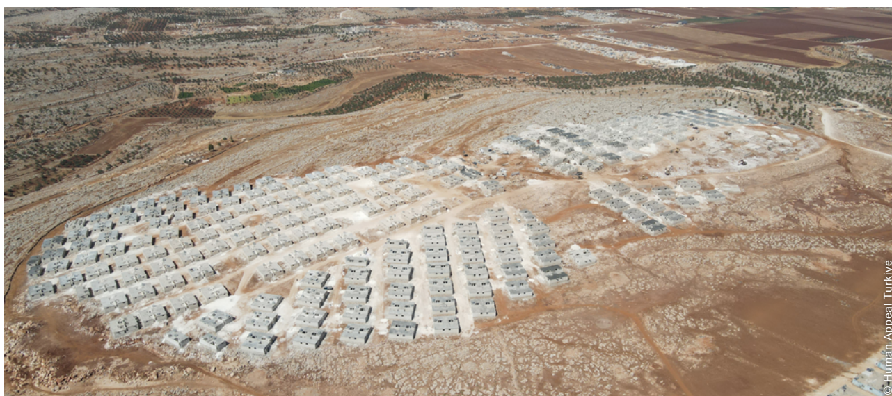
1,000 shelters were built on the site for IDPs affected by the earthquake. The project had already targeted families displaced by the Syrian crisis, but was rapidly adapted following February 2023. The site was chosen with local authorities and due to the proximity to other existing communities, ensuring it would not be isolated.
