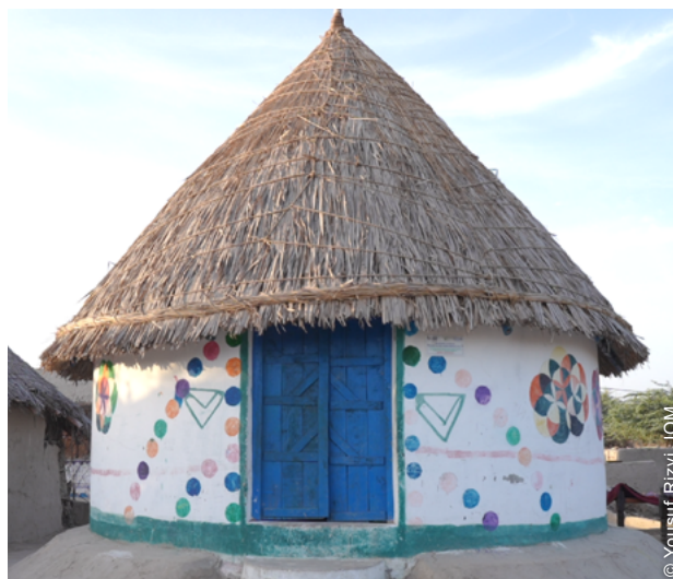
The design choices, including the circular shape and conical roofs, helped reduce the amount of bricks and contributed to budgetary savings.
