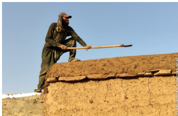
The project also trained 83 local masons in vernacular construction techniques.
