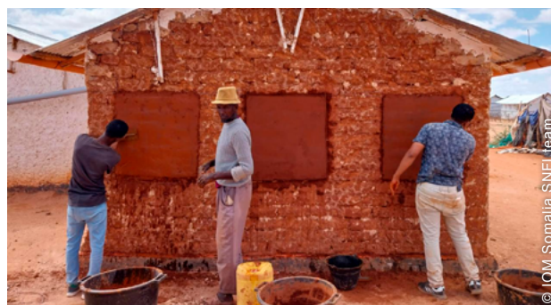
Training on eathern construction techniques, including plastering, was key.
