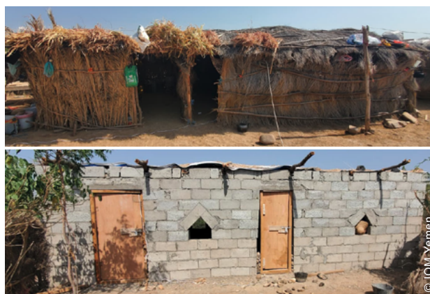
The project supported families across sites to repair or upgrade their shelters.
