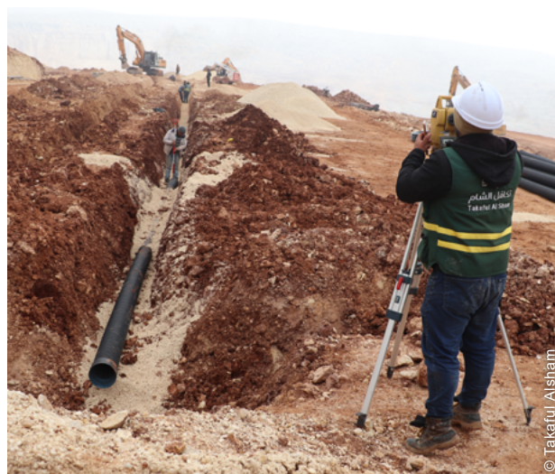
Water and sanitation services were installed to make the site habitable.
