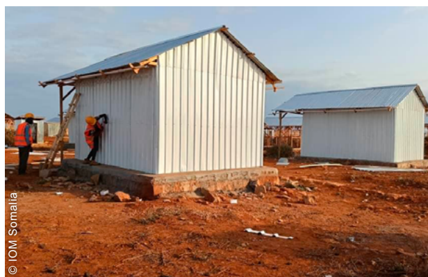
Because of budgets and government requirements, most shelters in the Barwaaqo relocation site were built with CGI sheet cladding for the walls.
