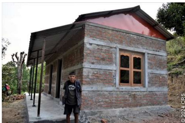
Multiple housing typologies and construction techniques were adopted, based on owner's preference, material availability and local context.
