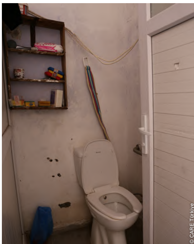
Works also focused on accessibility improvements for people with disabilities.
