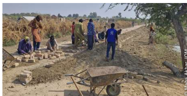
The project also implemented community works such as pathways, using cash for work, which proved essential to improve accessibility especially during floods.
