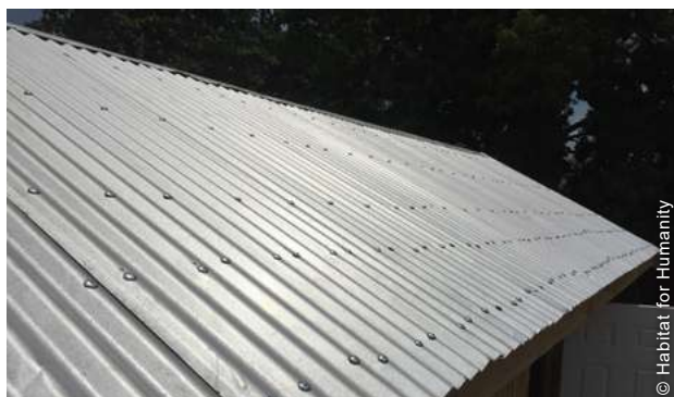
The correct use of roofing nails was implemented to prevent wind uplift.
