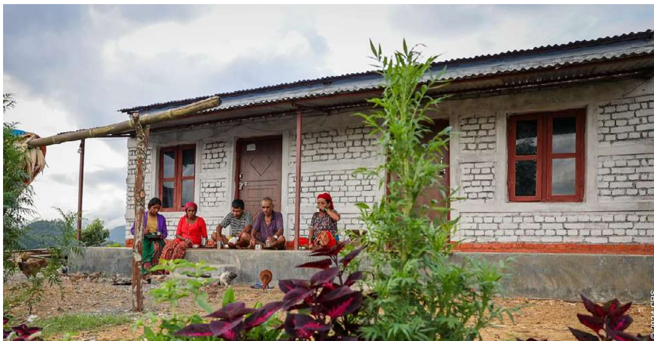
The project provided multisectoral support to households who, after six years from the earthquake, still hadn't been able to access reconstruction assistance.
