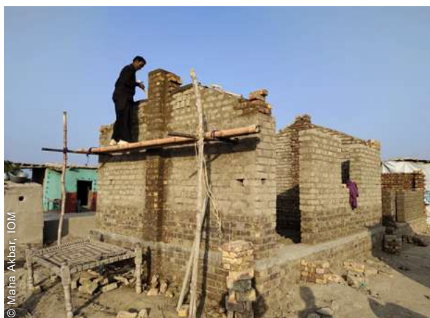
During the first phase of the project, stabilised mudbrick shelters were constructed, but were later discontinued in the subsequent phases.
