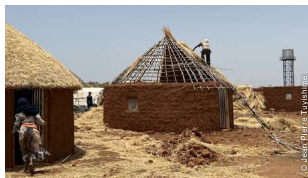
The roofs used local wood, the frame was assembled on the ground and completed with thatch to waterproof and improve thermal comfort.
