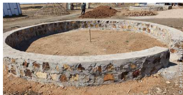
Raised reinforced foundations and backfilling protected from flooding.
