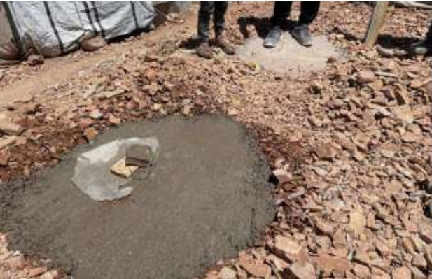
B - Concrete foundation pockets/slabs
