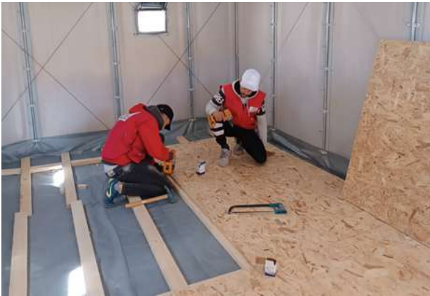
D - Installation of OSB wooden flooring platforms
