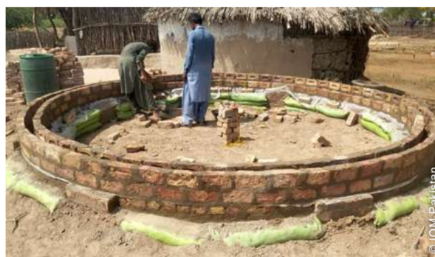
Pier foundations with sandbag infill were introduced following project extension.
