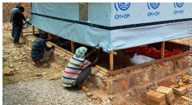
The incremental upgrading process encourages participation of the households in the construction process and promote livelihood opportunities
