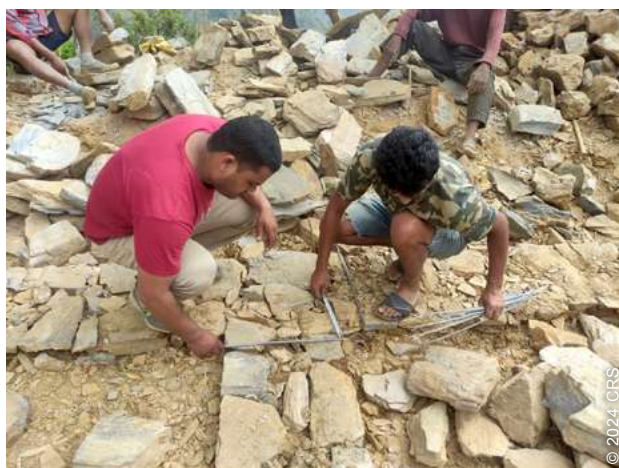
Several technical solutions were identified for improved earthquake resistance, including for traditional construction techniques, such as including galvanised iron wires in stone masonry with mud mortar.
