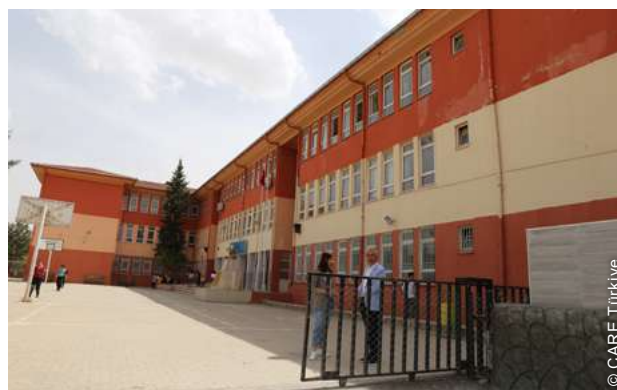
Beyond shelter rehabilitation, the program renovated 150 communal buildings such as schools and health facilities, using an area-based approach.
