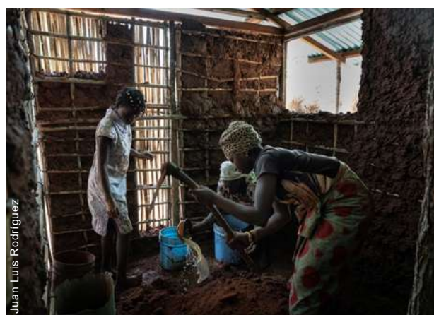
Women taking part in wall-mudding for a shelter construction in Mozambique
