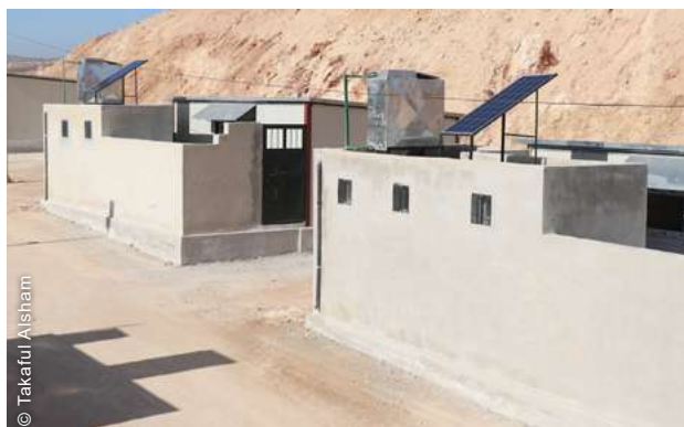
Solar panels and water tanks were installed over the sanitation blocks of the units. Site level interventions also included a water network and waste bins.
