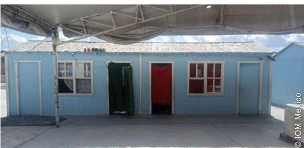
To increase comfort, safety and habitability, the organization provided timber shelters to accommodate part of the migrant population at the centre.
