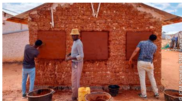
Training on earth construction techniques, including plastering, was key.
