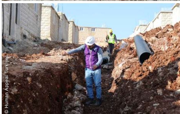
Following site preparations, the organization focused on the main services, including drainage, water and sewer systems, before shelter completion.
