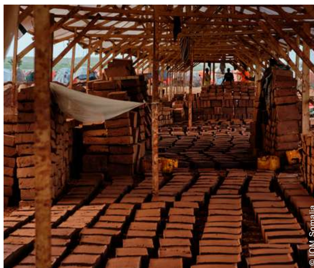
Earth-based construction, and primarily adobe (mudbricks), was promoted but could not always be adopted at scale due to limited familiarity of the techniques and perception barriers.
