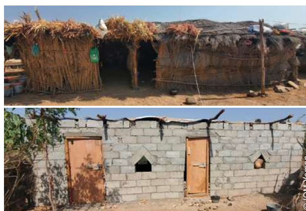
The project supported families across sites to repair or upgrade their shelters.
