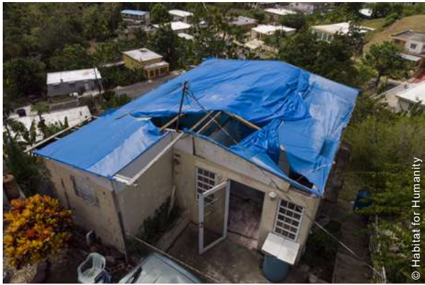
Storm-affected houses were temporarily covered with tarps prior to the repairs.
