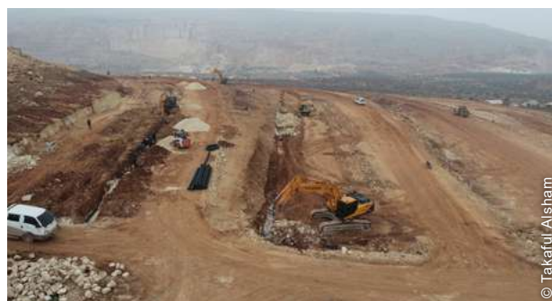
Sewer pipes were installed along the main roads of the new settlement.
