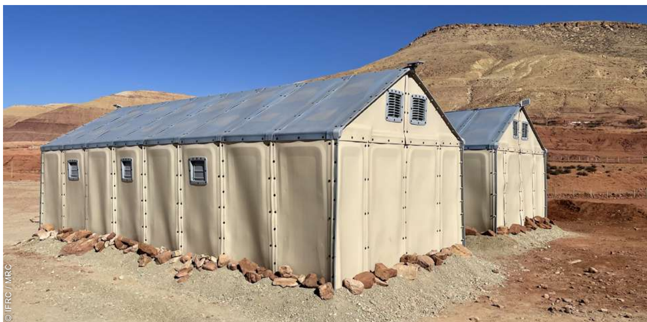
The imported shelter units, which costed around USD 1,765 including transport to Morocco, had to be adapted to the mountainous conditions, with add-ons and adjustments that costed on average an extra USD 1,000 per unit. One of the adaptations had to do with safe anchoring of the foundations against the wind.
