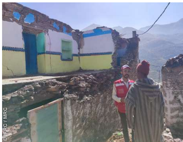
In hard-to-reach areas, humanitarian actors complemented the government reconstruction efforts. This project targeted families who needed a transitional solution before the reconstruction could be completed.
