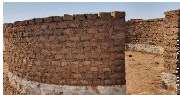
The adobe walls provided good thermal insulation and security.
