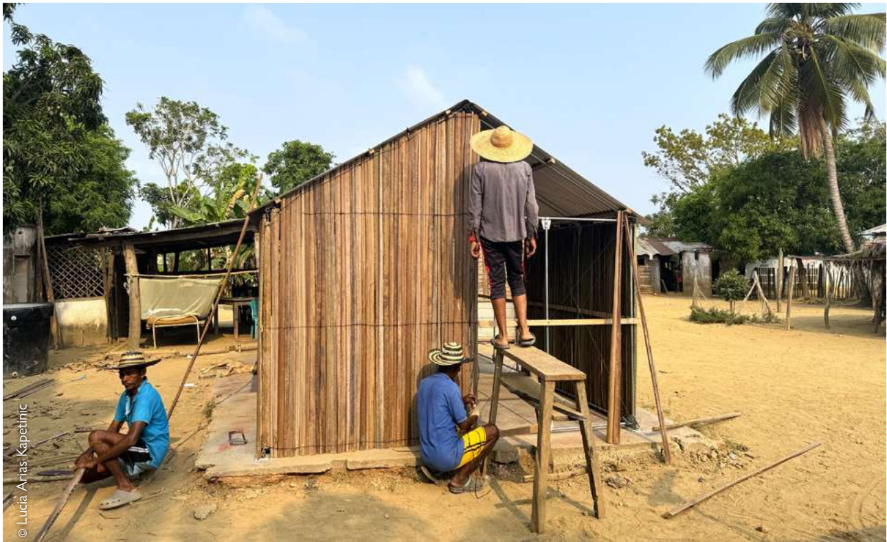
Francisco Luna's new home under construction in El Chopa, Colombia, March 2024, replacing one that collapsed twice.
