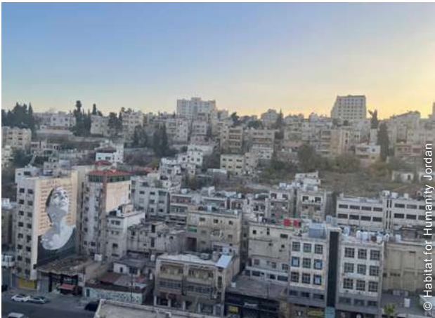
The project rehabilitated homes and public facilities in urban areas of Amman, serving both Syrian refugees and local Jordanians.
