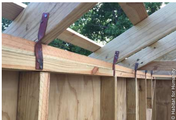
Model houses adopted hurricane-resilient features such as metal straps.
