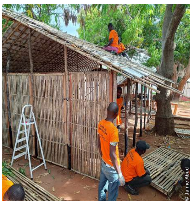
Prototypes were built during BBB trainings using vernacular techniques.
