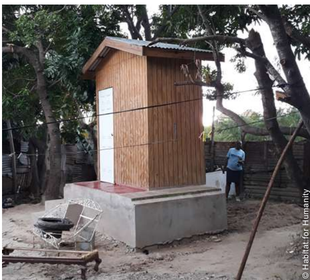
The program also included a WASH component, including the construction of elevated flood-resilient latrines, which were implemented through contractors.
