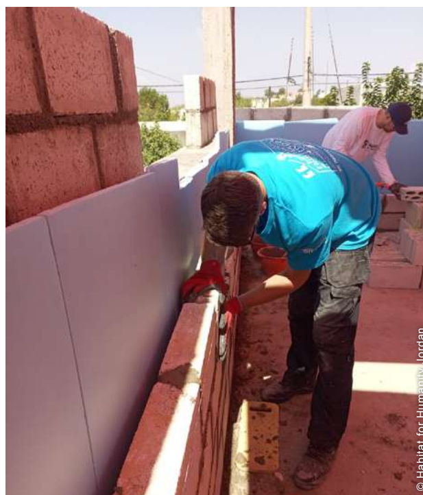
Insulation panels were installed where possible to improve indoor comfort.
