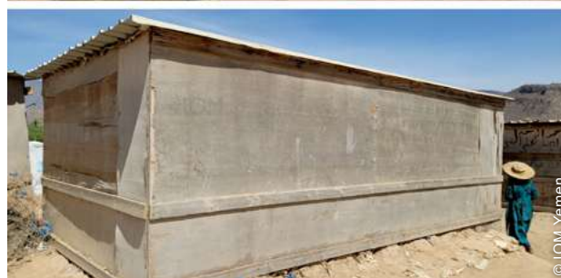
The support was also used to protect plywood from heavy rain with metal sheets.
