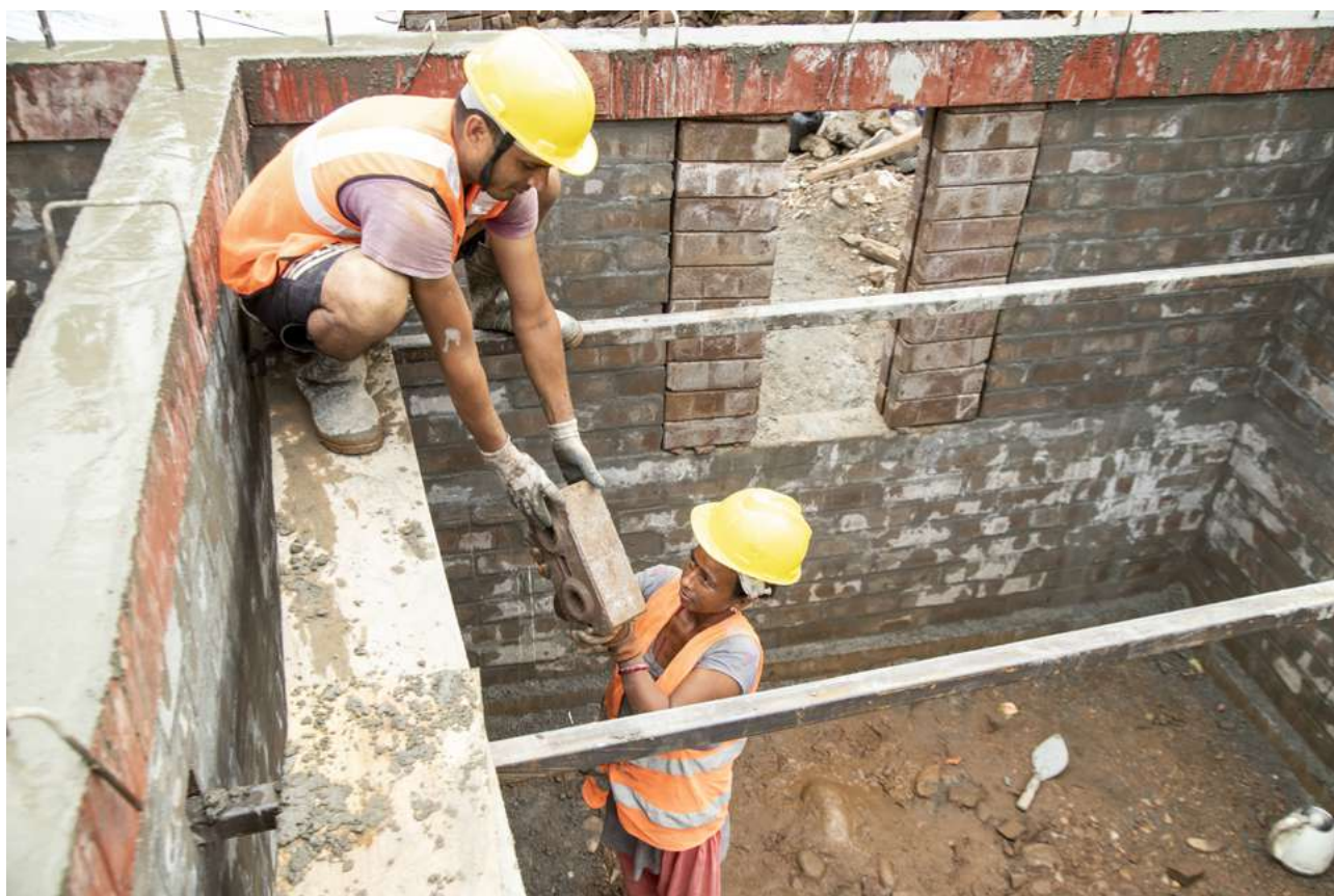
Shelter construction in Nepal.
