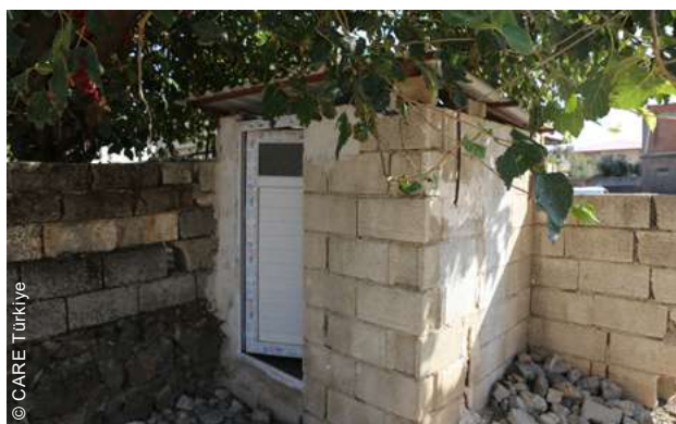
Rehabilitation works included WASH facilities and kitchens, and were implemented with a cash-based modality in two tranches.
