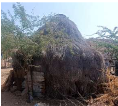
Displaced families in Yemen lived in different types of makeshift shelters, built using locally available materials and based on cultural and contextual factors.
