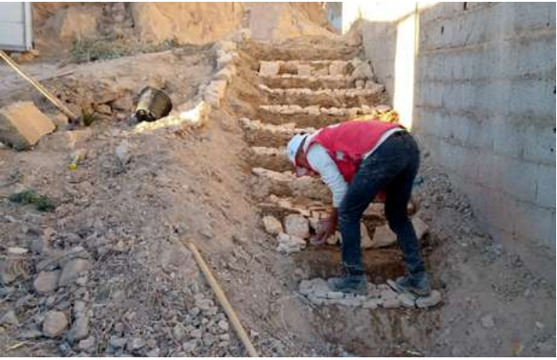
E - Construction of ramps and adapted site layouts
