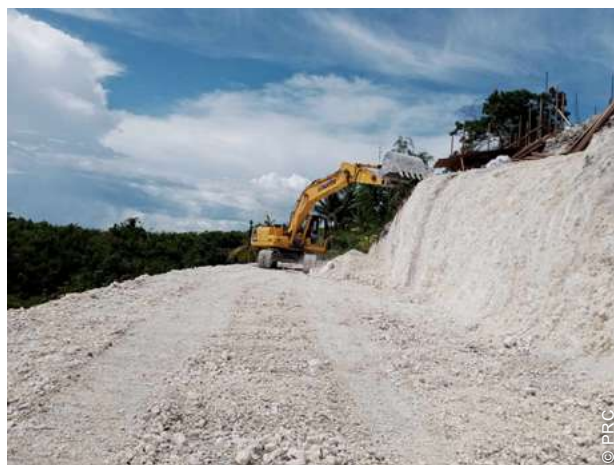
Due to the terrain, unforeseen presence of large boulders and varying soil conditions, site works required heavy equipment and longer than expected.
