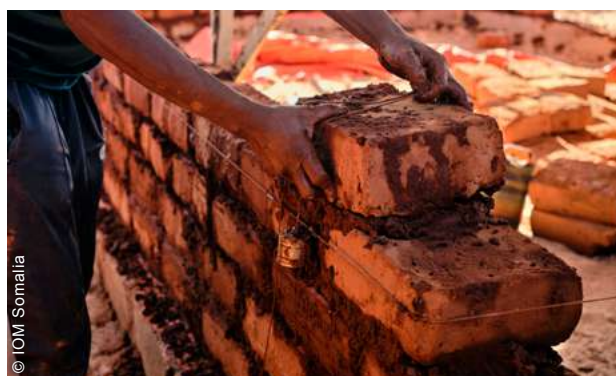
Mudbricks were used to upgrade the walls of emergency shelters.
