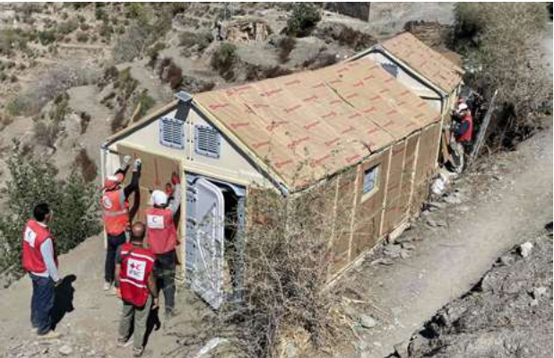
A - Insulation using rockwool covered with tarpaulin and protective layers
