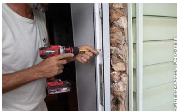
Common repairs included insulation and replacement of doors and windows. Beyond the vouchers, the project provided cash to cover for the labour part.
