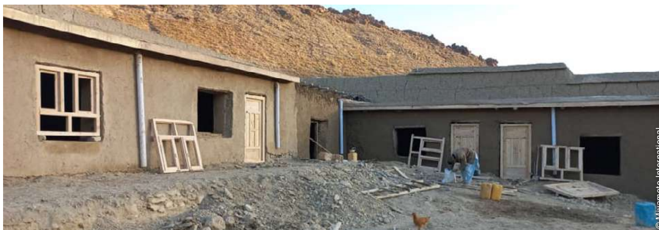
The importance of the compound life was understood and supported by the project, which included boundary walls and clustered configurations in the reconstruction.
