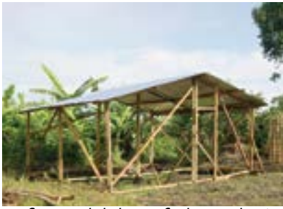
Structural skeleton of a house, showing cross-bracing
