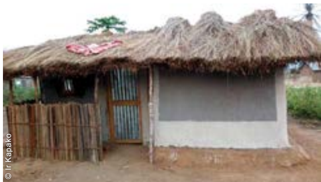
Communities actively participated in the design process. Thanks to their inputs, the shelters were expanded and a shaded veranda was added.
