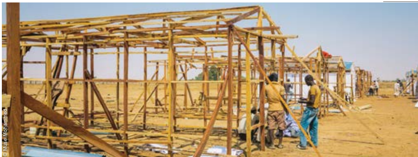
The shelters were built by contractors, with the condition that they hired workers locally including IDPs, who received on-the-job training.
