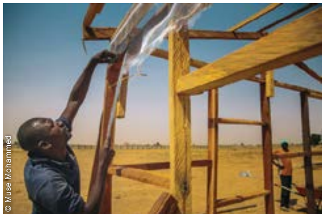
Shelters included specific details, such as mosquito nets in the open gap beneath the roof, which was intended for ventilation.
