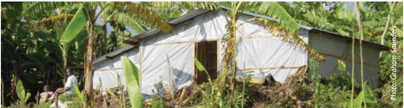
Sample of a temporary house
