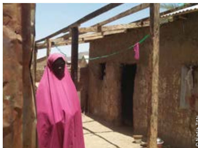
In some cases carpenters helped vulnerable members of their communities to rehabilitate their houses.
