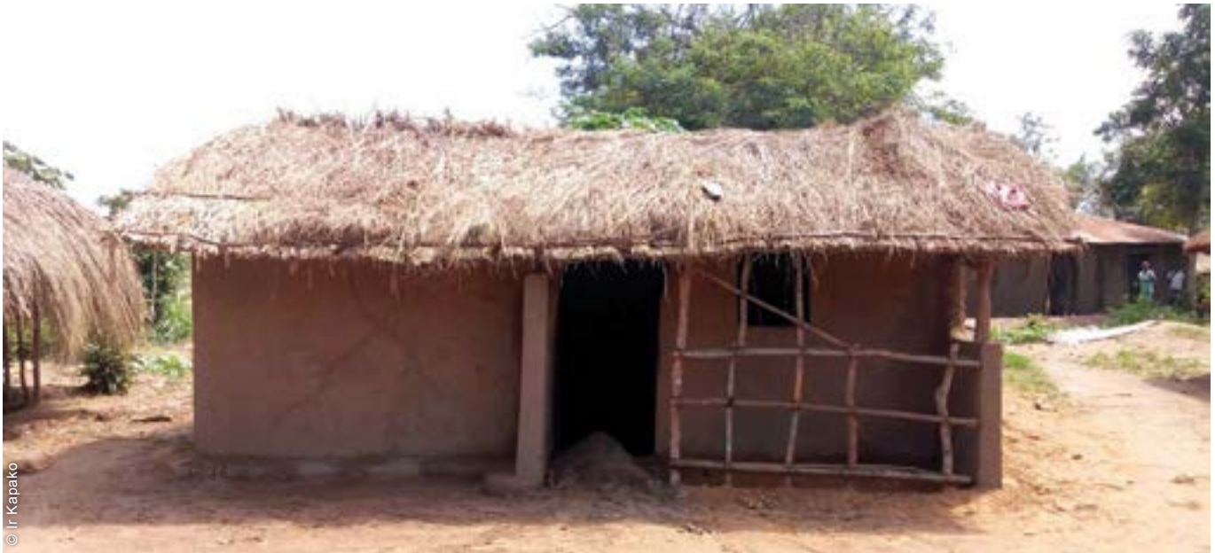
Shelters were cost-effective, as materials were locally available and labour was provided by the affected families themselves.
