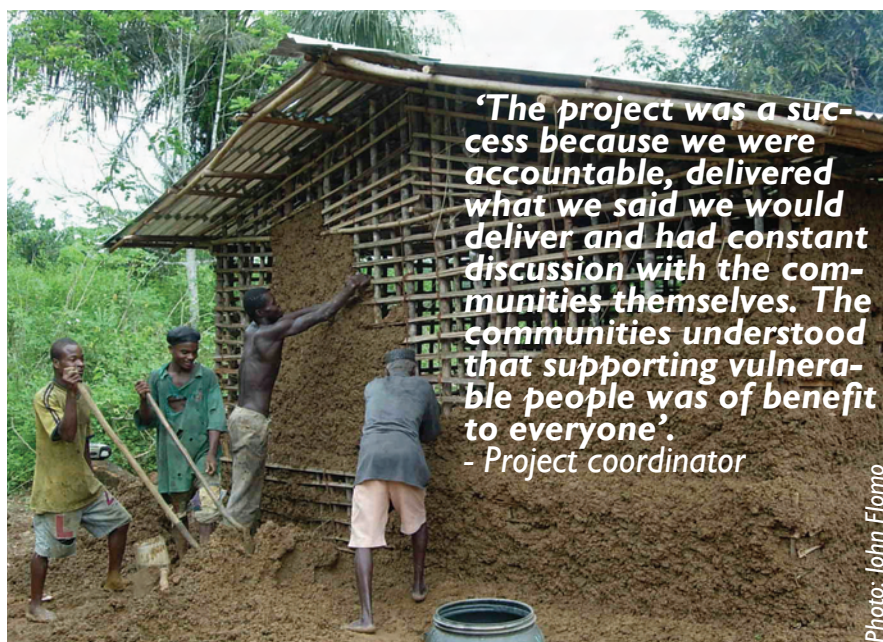
Traditional shelters under construction
