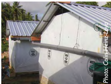
Shelters built with tanks for rainwater harvesting
