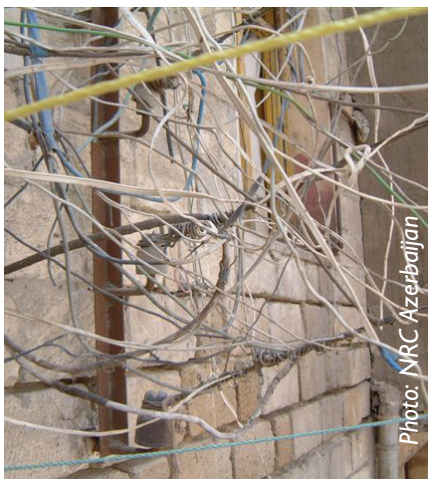
Wiring before upgrade
