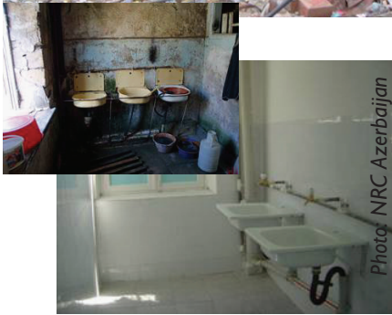
Bathrooms before and after upgrade
