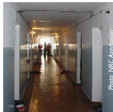
Corridors before and after upgrade
