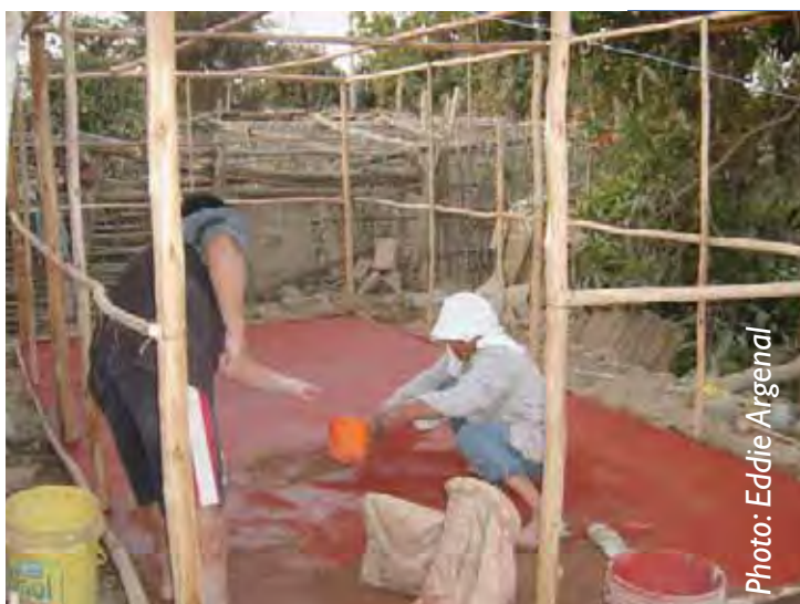
Making the concrete floor slab
