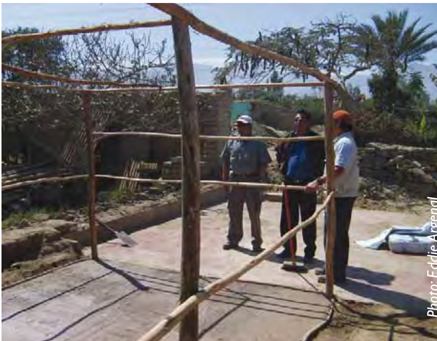
Round poles, not sawn timber, were used
