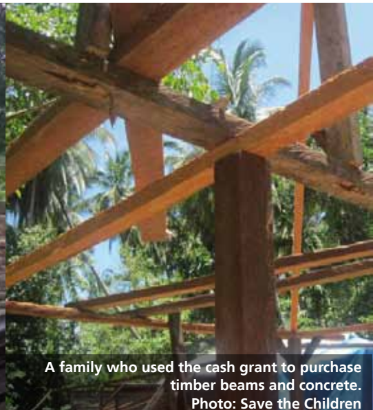
House for 9 people under construction in the foreground. Photo: Save the Children
