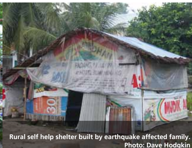
200 USD "transitional shelter" of disappointing quality built by an international organisation. Photo: Dave Hodgkin
