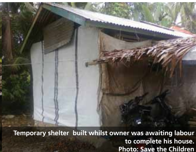
Many materials could be salvaged. Cash grants allowed people to pay for materials and labour according to their needs.
