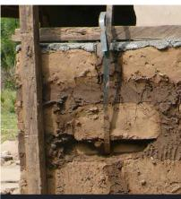
Fixing the roof to the wall: a wood block has to be placed between the mud bricks and strapping to stop it tearing through the wall.
