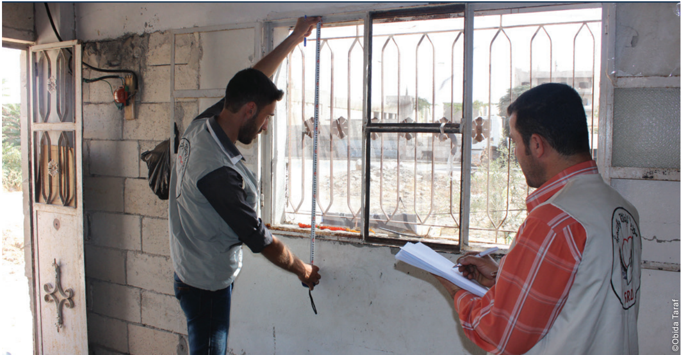
The project included repairs and upgrades to walls, floors, ceilings, doors and windows and installation of wiring, plumbing and latrines.
