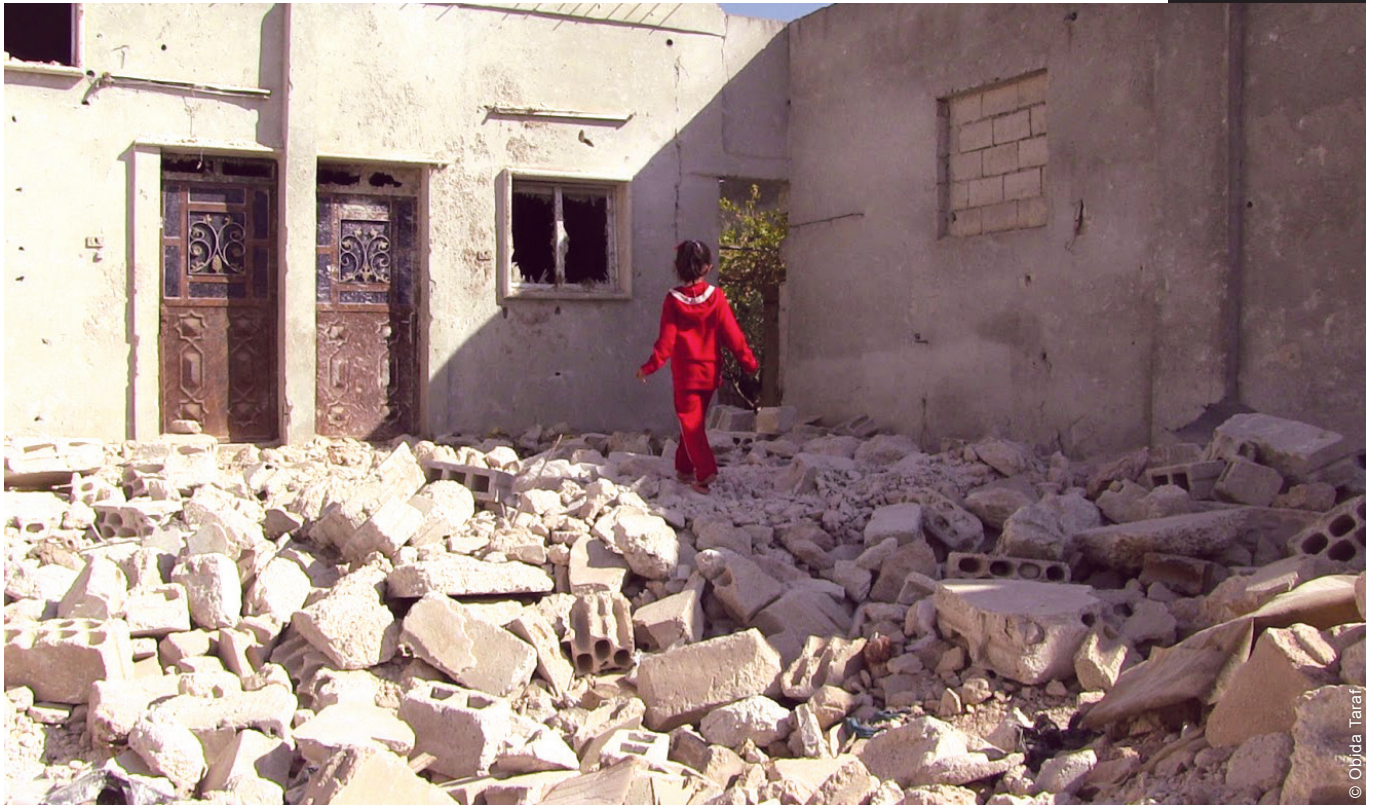
The extent of the damage to private properties, particularly the housing stock, has reached extreme levels within the Syrian Arab Republic. Before the rehabilitation of each house could start, the technical team had to check the local conditions and structural integrity.
