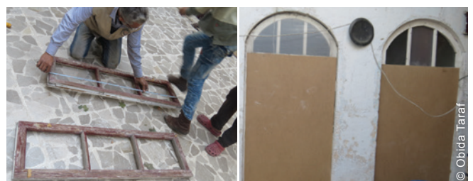
Repairs included the replacement of window frames or sealing off of openings.
