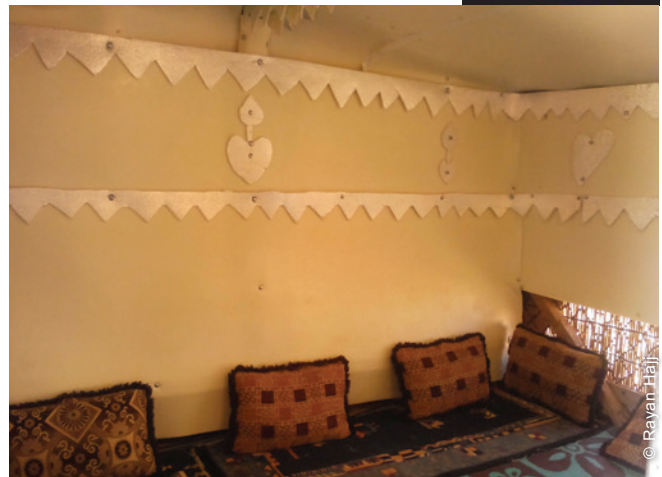
The insulation foam was to be applied to both walls and ceilings, and in some cases people were creative and made decorations out of the same material.
