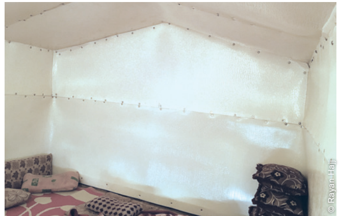
The foam was applied to walls and ceiling, while mats and pillows were used to insulate the floor. This achieved a full insulation of the shelter, which ensured a significant reduction of the heat loss during the winter, as well as good performance during the summer.
