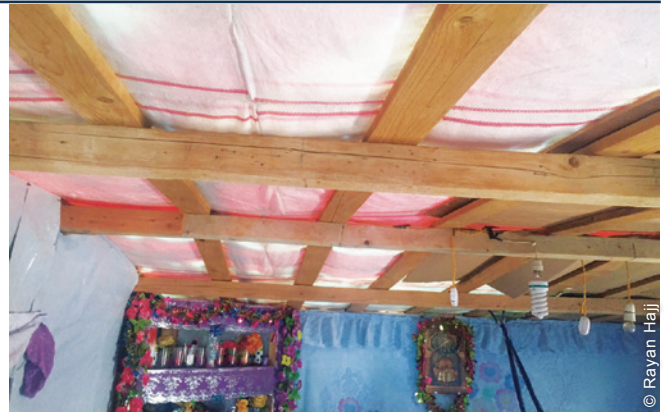
Before installation of the insulation kits, poor quality plastic sheeting and other temporary materials, such as cardboard, were commonly used in most of the shelters targeted by this project.
