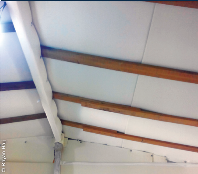
People installed the insulation foam to reduce the heat loss, which generally tends to be higher through the ceiling/roof and the floor/ground.
