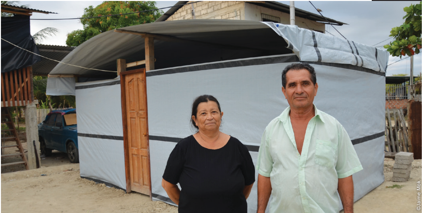
The project provided earthquake-affected families with emergency shelter kits and trainings at the community level, so that they could be better able to build shelters.
