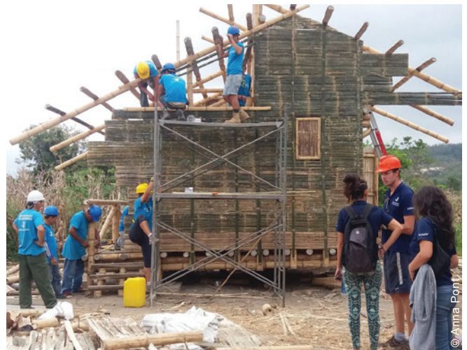
Humanitarian organizations built transitional shelters made of local bamboo, often with the help of volunteers from local NGOs.
