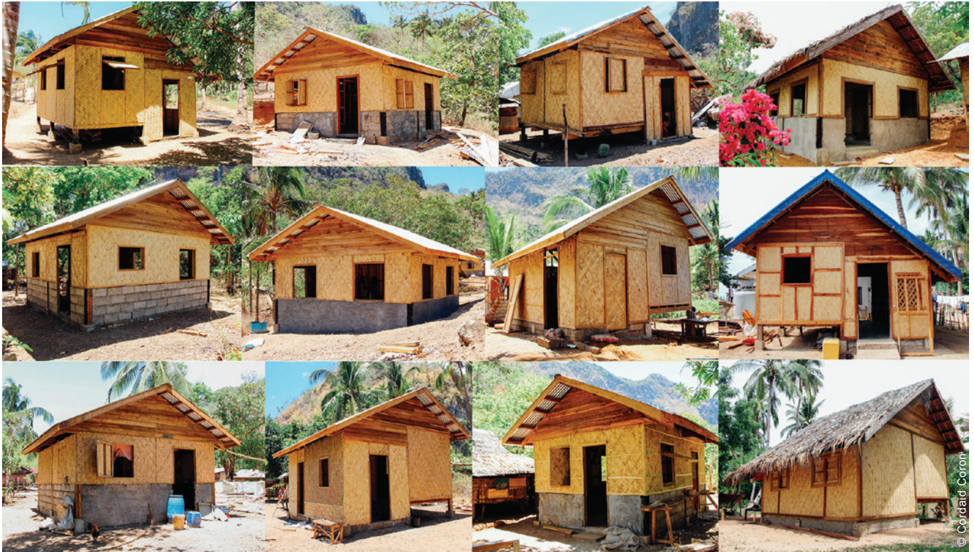
Examples of the houses built through the programme. Each household was free to adopt a different design, and manage the construction directly.
