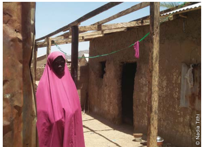
In some cases carpenters helped vulnerable members of their communities to rehabilitate their houses.
