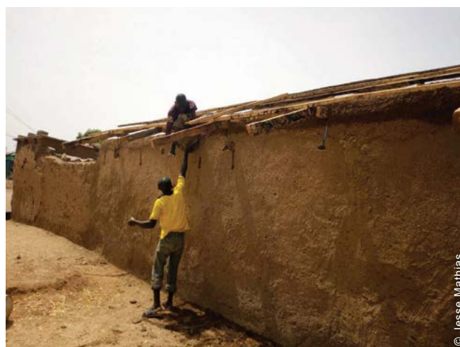
Families were able to repair their entire house, in some cases even expanding the original size. This also supported family reunification.
