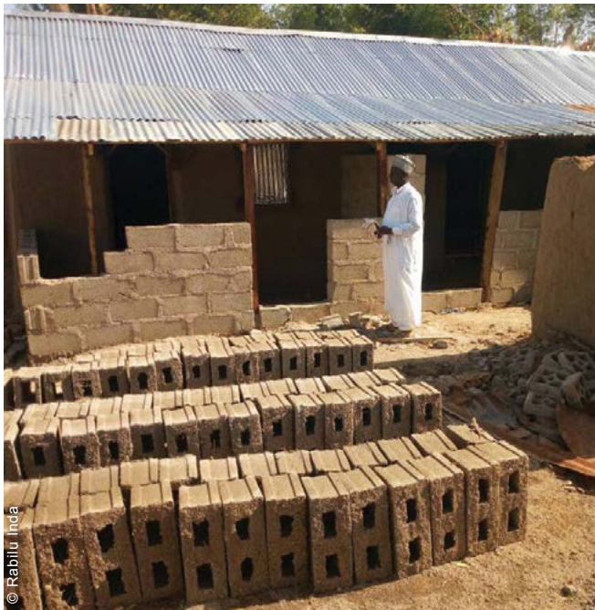
Beyond shelter repairs, the project also included livelihood and community infrastructure rehabilitation components.
