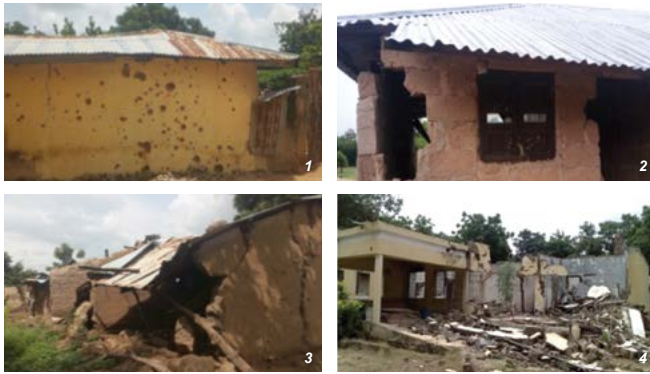
Damage was categorized in four groups. 1) Bullet holes on the external walls but not penetrated inside; hairline cracks in very few walls; fall of small pieces of plaster only. 2) Doors and/or windows need to be replaced, damage to brickwork 10%. 3) Failure of structural elements, damage to walls 25%. 4) Completely damaged with bullet holes, serious failure of walls; partial structure failure of roof and floor.
