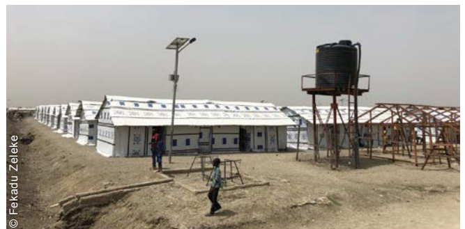
The project rehabilitated a sector of the Malakal PoC through a phased approach.
