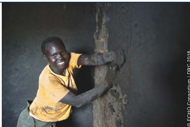
The project engaged local youth throughout the construction process. In some cases, the rendering phase presented some challenges for the beneficiaries.
