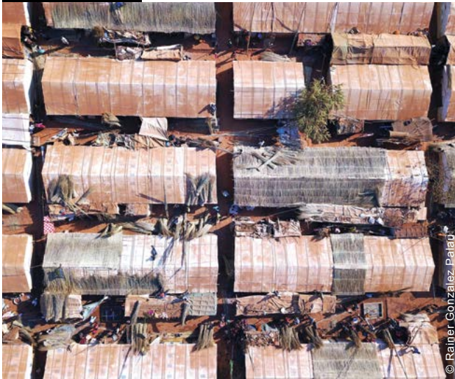
One of the upgrades consisted of adding a layer of dry elephant grass to rooftops to increase protection from the elements, improve ventilation and lower inside temperatures.
