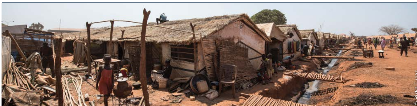
People on the site lived in communal shelters. The project upgraded the walls and roofs to extend their lifespan by protecting the plastic sheets.
