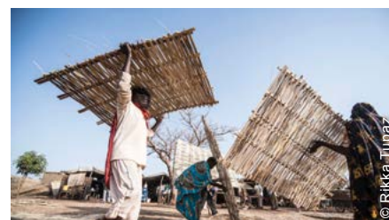
The project engaged local traders and trained beneficiaries on the upgrades, which included the addition of grass to rooftops and bamboo-thatched walls.
