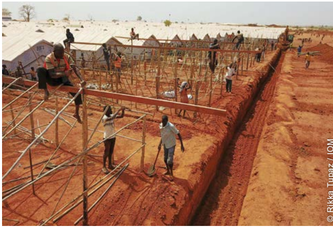
Shelter construction, upgrade and site rehabilitation were common activities conducted in PoCs in 2017–2018.
