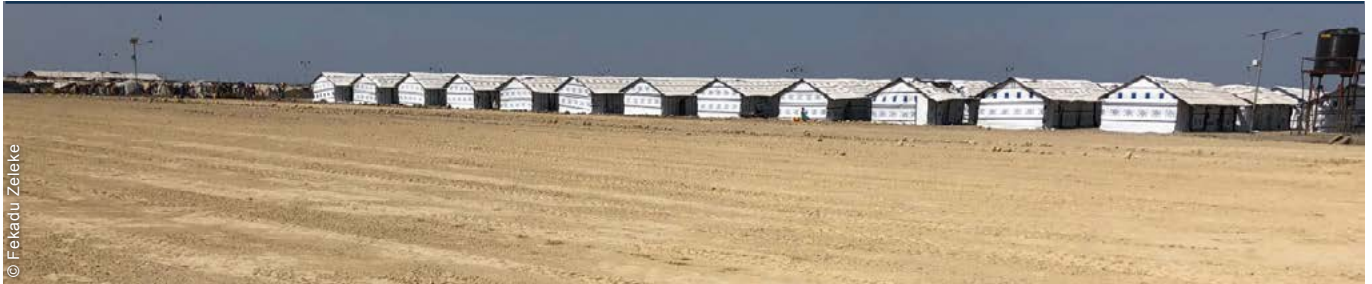
Priority activities in the rehabilitation included backfilling, ground levelling, reconstruction of drainage and rehabilitation of secondary roads, as well as reorganization of the space to improve access to services.
