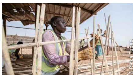
The project engaged local traders and trained beneficiaries on the upgrades, which included the addition of grass to rooftops and bamboo-thatched walls.
