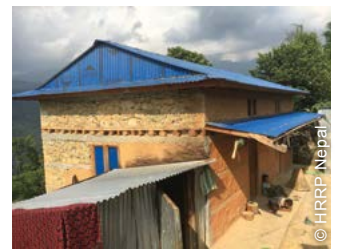
Government grants were used to rebuild a variety of different housing typologies. From load bearing brick masonry and reinforced concrete (above-left) to timber frame and stone masonry (above-right).
