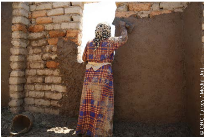
It was challenging to involve women in the construction, but the project succeeded in engaging some of them throughout implementation.
