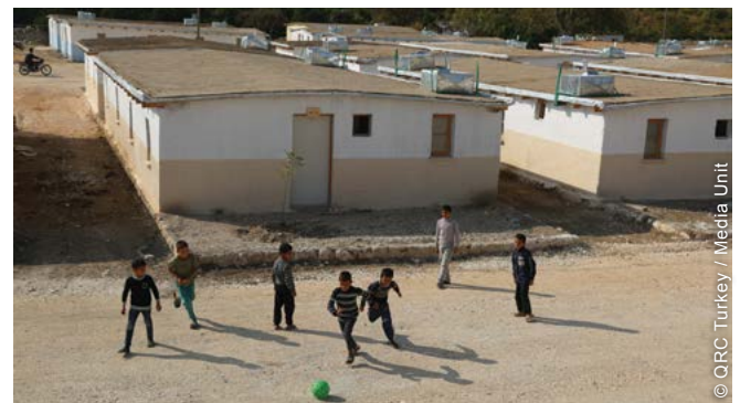
Displaced households were involved in the design of the houses.
