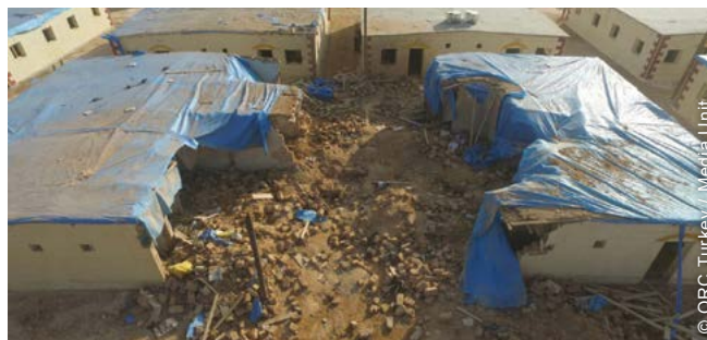
One site was hit by an air strike, highlighting the security risks in the project areas.
