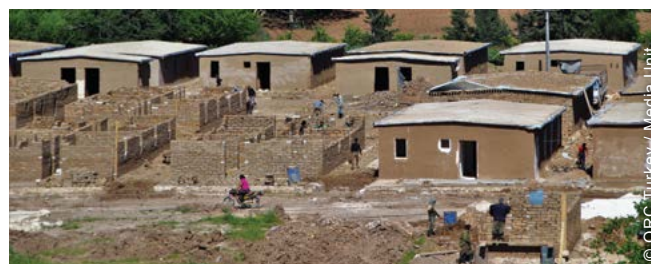
The project had a low environmental impact thanks to the use of mud bricks. Settlements were built as transitional and could be dismantled after the conflict.
