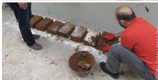
A ToT on local building cultures was organized in Turkey in partnership with an international consultant. Adobe was selected as the material for the houses.
