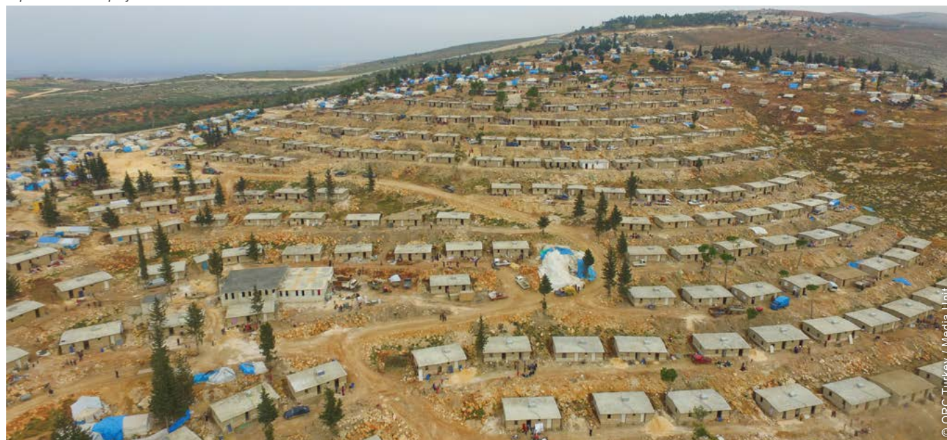
The project was implemented in five different locations close to the Turkish border in Syria. Soil for bricks was sourced in abandoned hills and holes refilled after extraction.
