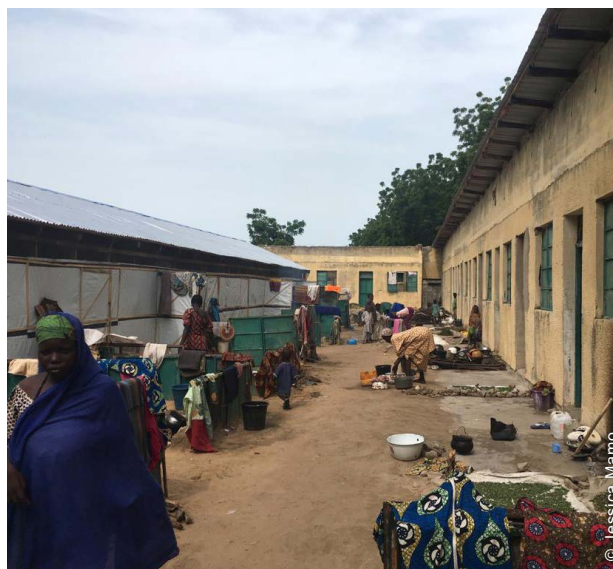
Existing buildings on the site were rehabilitated and partitioned (right) to provide additional shelter in the camp. Partitioned communal shelters (left) were also constructed due to the lack of space for individual family shelters.
