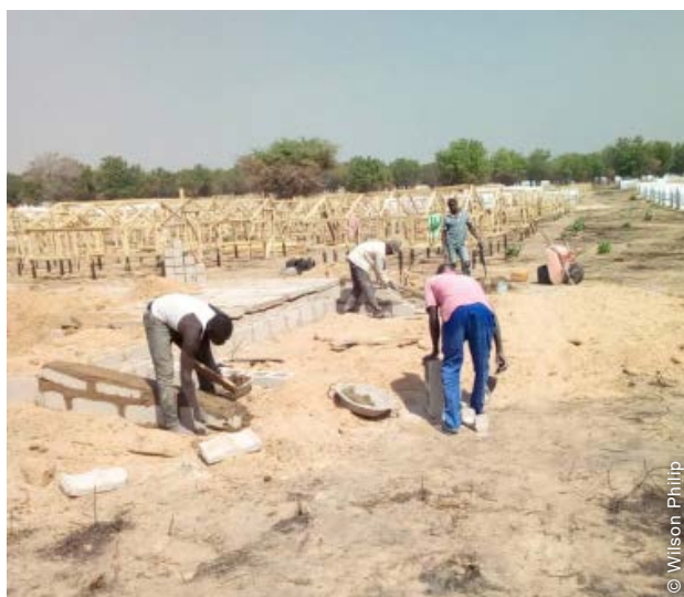
Shelter and latrine construction commenced in October 2017 in preparation for the anticipated relocation date of January 2018 (which was later brought forward to mid-December 2017).
