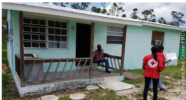
Homes outside of Freeport, the main city on Grand Bahama, are typically timber framed or concrete block single story structures.
