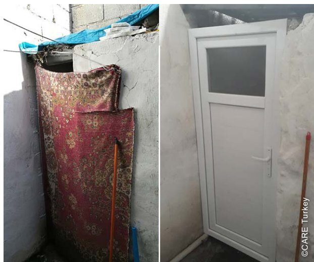
Before and after: Installing doors to improve protection, security and weather-proofing was a priority intervention.
