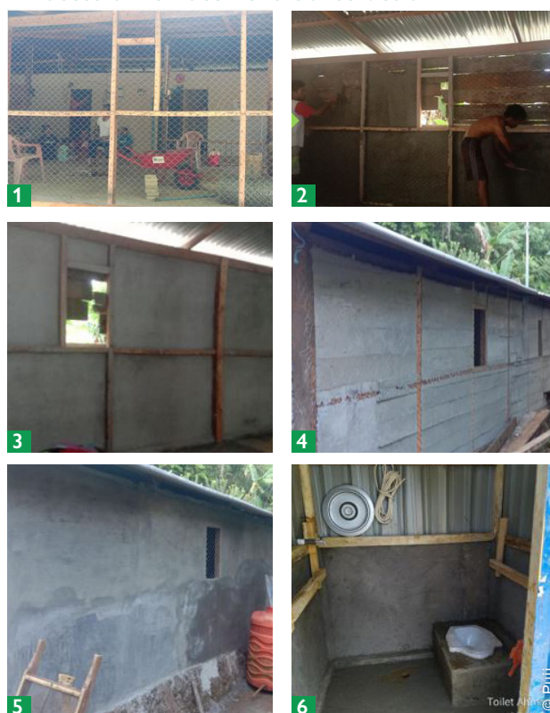
1: Construction training; 2: First formwork; 3: Inner plastering; 4: Outer plastering; 5: Outer plastering completed; 6: View of a completed room.
