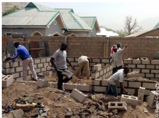
Construction of the permanent shelters using blockwork.
