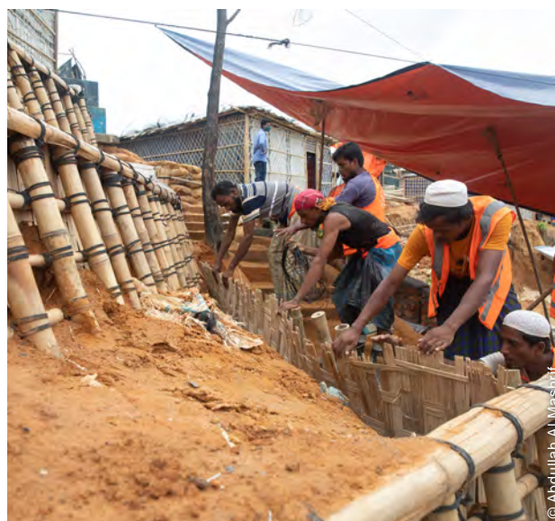
Site development work of reconstruction of bamboo slope stabilisation and access carried out by people engaged in Cash for Work, February 2022.
