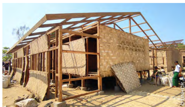
The reconstruction works included the replacement of the timber frame and bamboo cladding elements of the longhouse.
