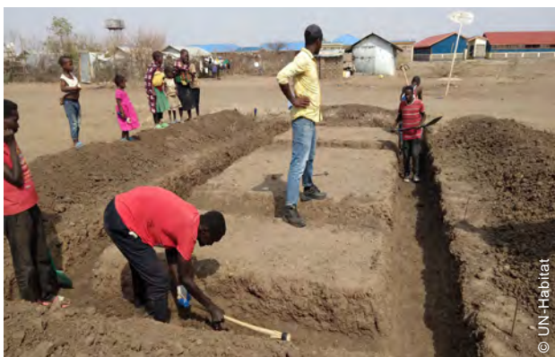
Images of the site construction activities. (Left) Excavations carried out by an artisan and two helpers for 2-3 days depending on the nature of the ground. (Right) Dressed stones were used for the walling of the superstructure.
