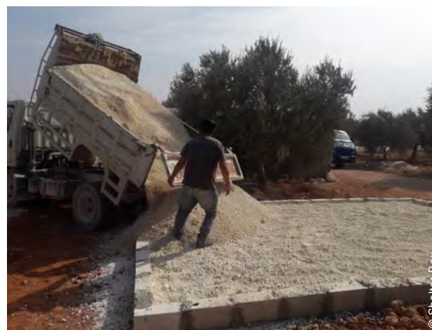
Tent leveling construction activities - (above) Building of the tent base perimeter with mortar blocks, November 2021. (below) Filling of the tent base with aggregate before the final cement layer, November 2021.
