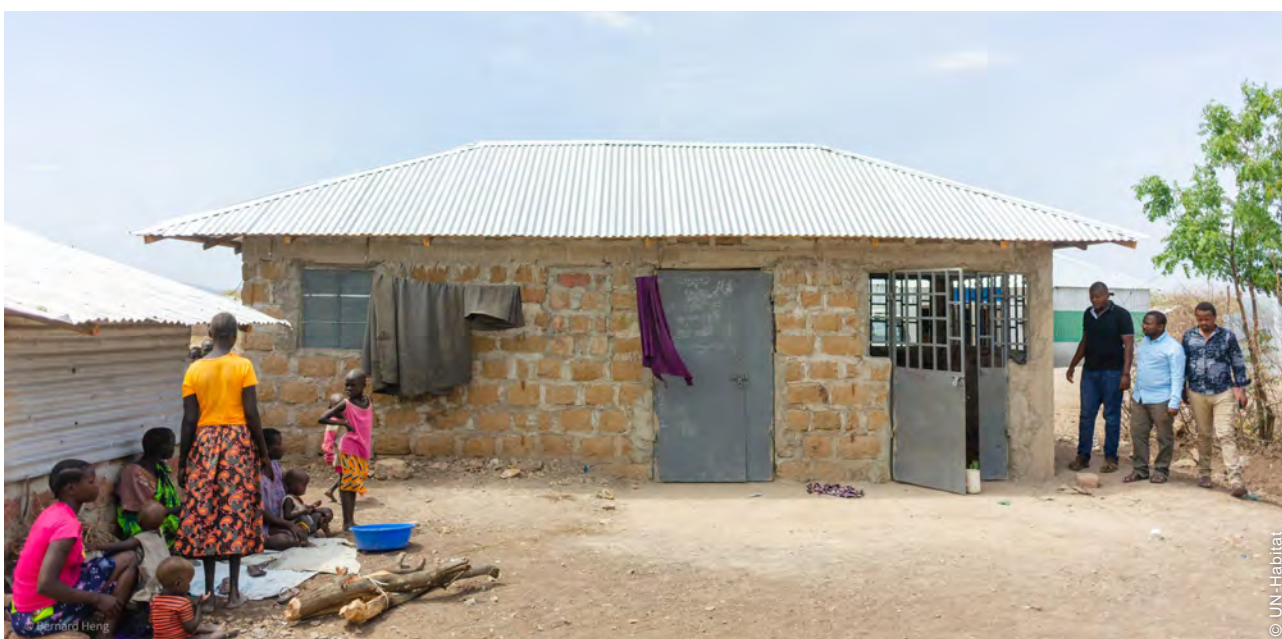
Families await the completion of their shelters. Passive cooling methods such as the use of natural turkana stone blocks and hollow blocks used in the construction controlled the temperatures inside the shelters.
