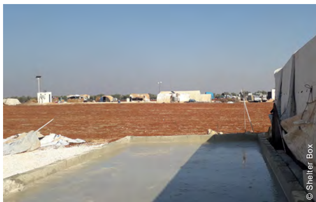
Cementing of the tent bases, November 2021. Size of the different tents were measured, and the tent bases were constructed according to the tent sizes.
