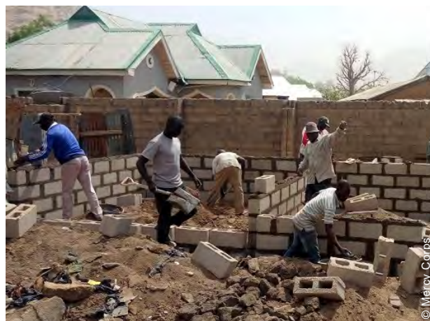
Construction of the permanent shelters using blockwork.
