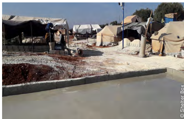
Cementing of the tent bases, November 2021. Size of the different tents were measured, and the tent bases were constructed according to the tent sizes.
