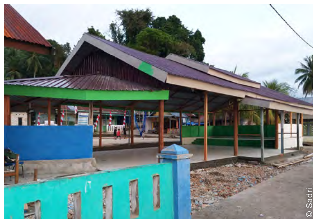
The Karampuang Village Community Hall before and after reconstruction. The project facilitated the community in Karampuang to renovate two Community Centres. The renovations were carried out using retrofitting and ferrocement methods. The renovation focused to improve better space, ventilation and lighting.
